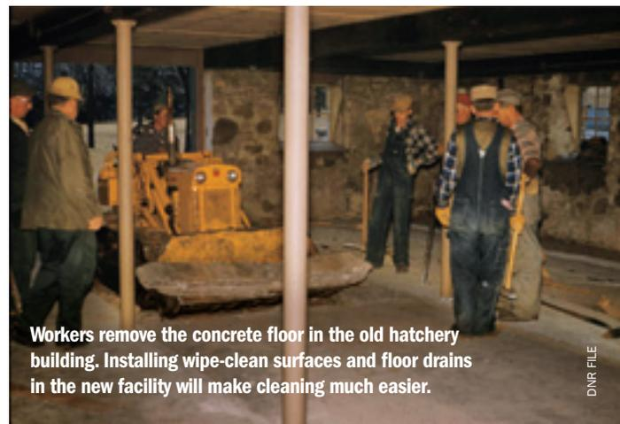
Workers remove the concrete floor in the old hatchery building. Installing wipe-clean surfaces and floor drains in the new facility will make cleaning much easier.
