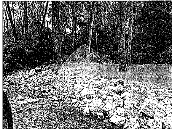
Photo: Typical view of the rip-rap stabilizations installed along 200LF of Pheasant Branch.
