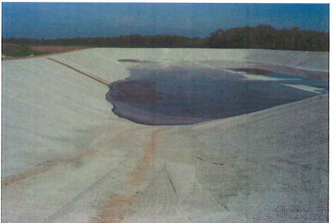
New pit being used.
