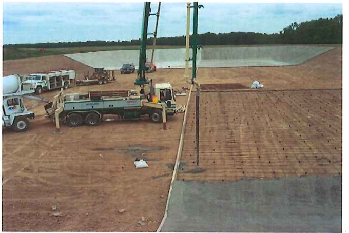
Concrete being poured in new pit.
