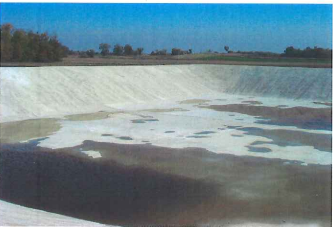
New pit being used.
