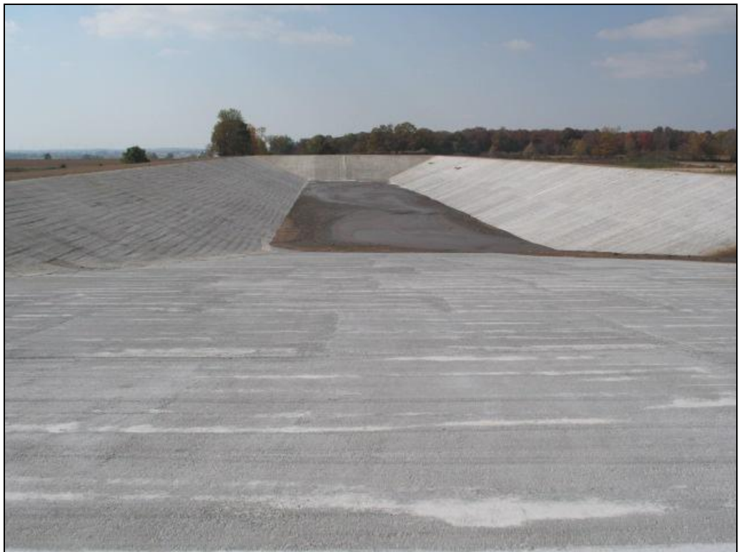
After - Looking West
