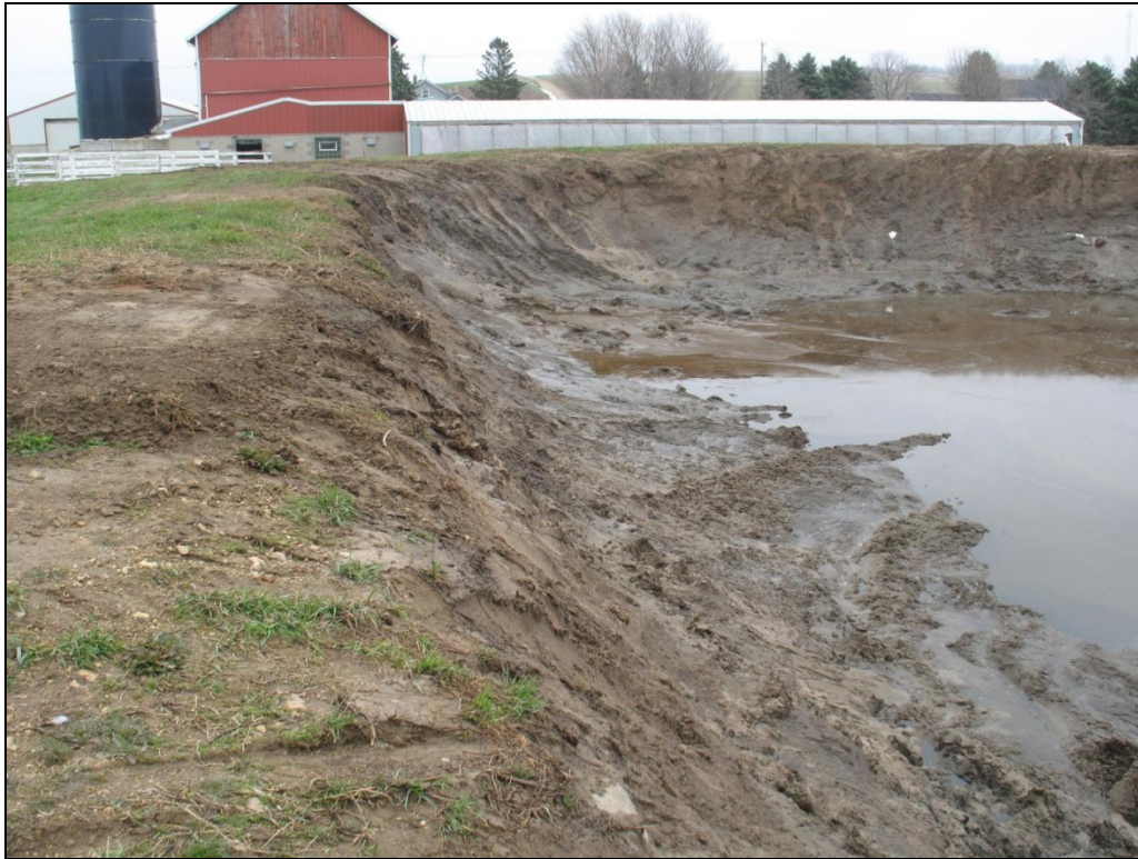
Before - Looking East
