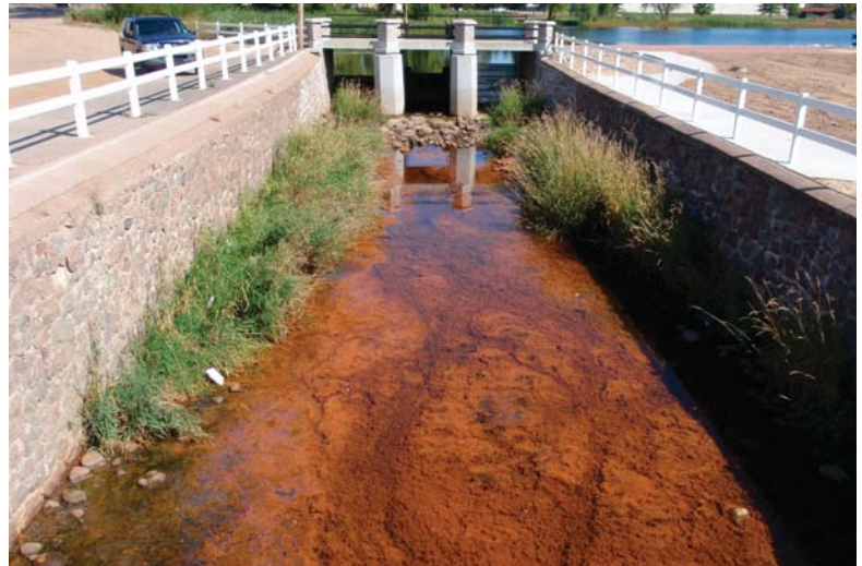
Springbrook Creek below the dam. This picture shows excessive iron bacteria, most likely caused by low flows due to drought and low discharge through the dam. Low flows with higher concentrations of groundwater (versus surface water) results in high iron concentrations, which precipitate out when exposed to oxygen at the water's surface.
