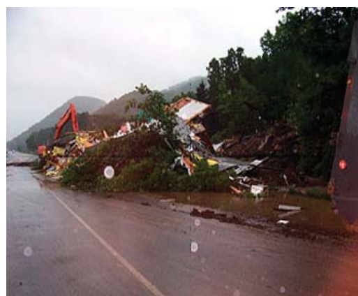
Mudslide that moved a house onto HWY 35 in Vernon County during August 18, 2007 flood. WDNR Photo
