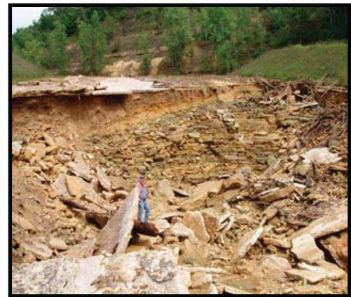
Aftermath of floodwater scour of the Runge Hollow Lake Dam emergency spillway on the North Fork of the Bad Axe River. August 23, 2007.
