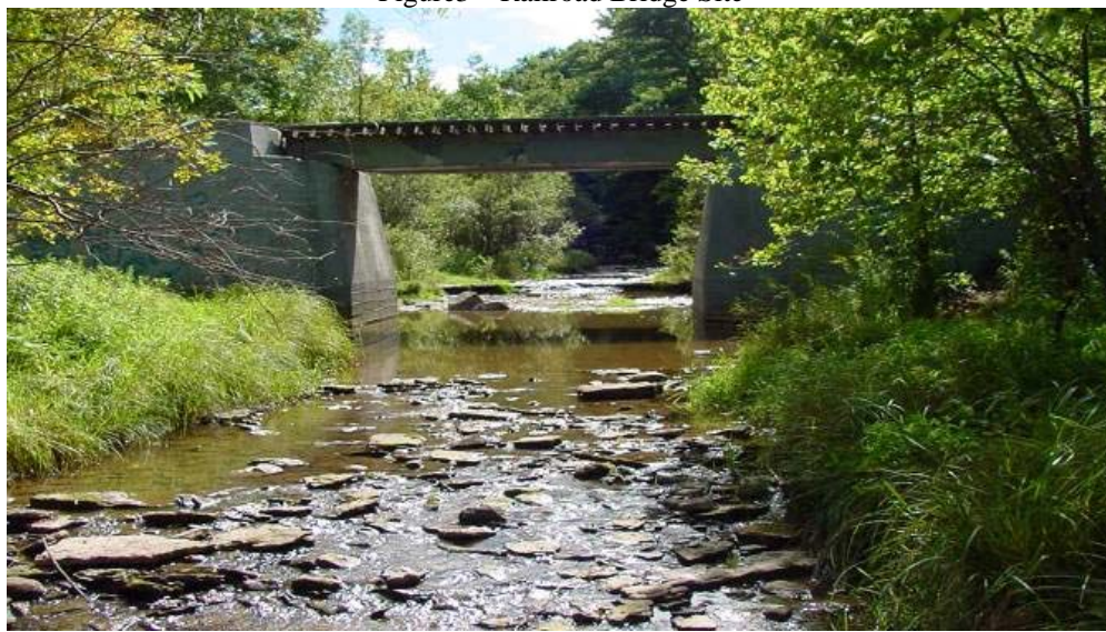
Figure3 – Railroad Bridge Site
