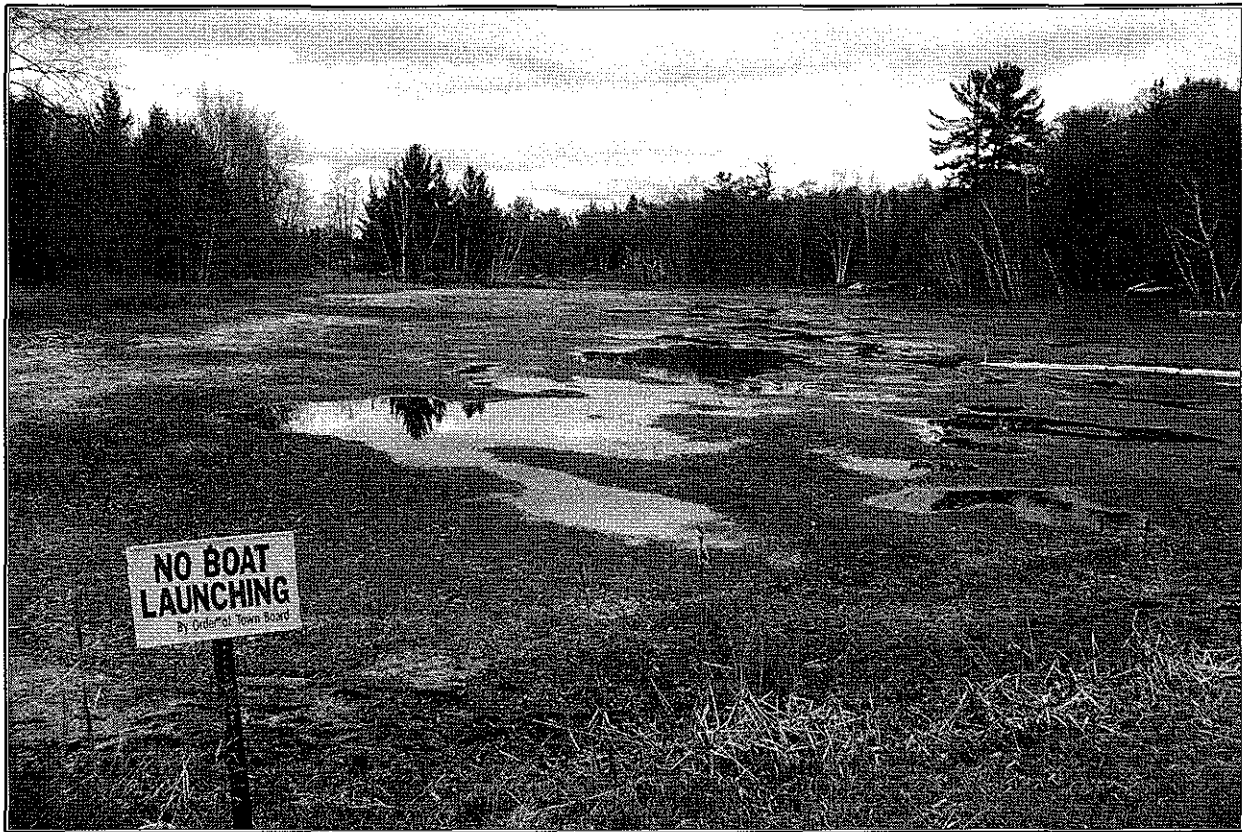
Figure 4. Five foot water level drawdown at the Beecher Lake Dam.
