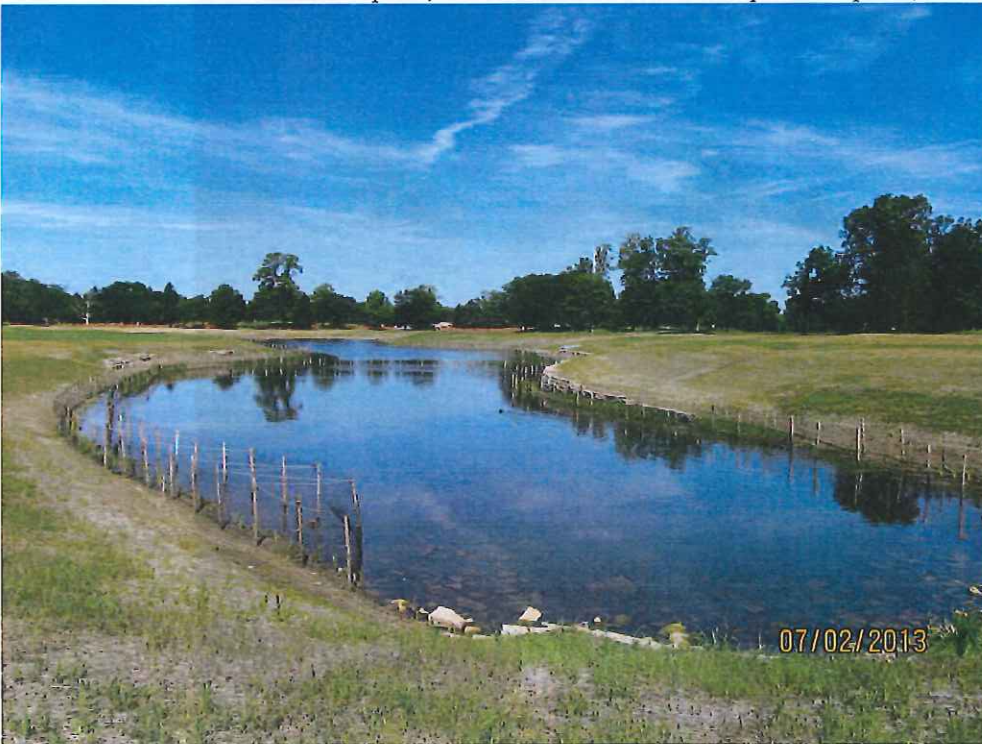
South Pond – Construction complete, exclusion fence & wetland plants in place, seeding completed.
