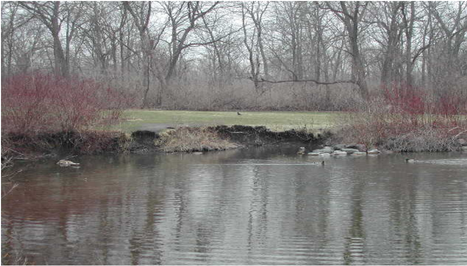
Spring Trail Pond. Shoreline erosion caused by resident (non –migratory) Canada geese and mallards.
