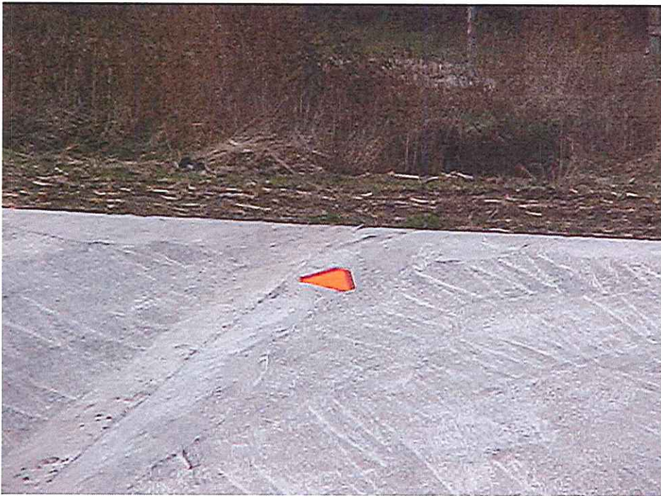
TRM Trapp Manure Storage Construction 2013
