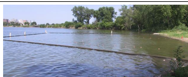
Fig. 8. Deflector boom system deployed at Bernie's Beach, June-August 2010-2011. (Photo: R. Lathrop, WDNR)
