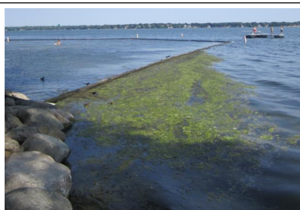
Fig. 6. Photo showing the deflector boom system preventing algae scums and other floating debris from entering the enclosed swimming area at B.B. Clarke Beach, June 2012. (Photo: C. Betz)
