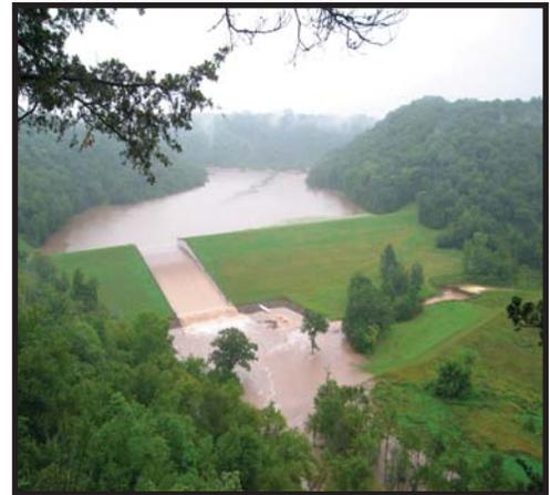
Floodwaters flowing over the emergency concrete spillway of the Springville Dam on the Springville Branch of the Bad Axe River. August 20, 2007.
