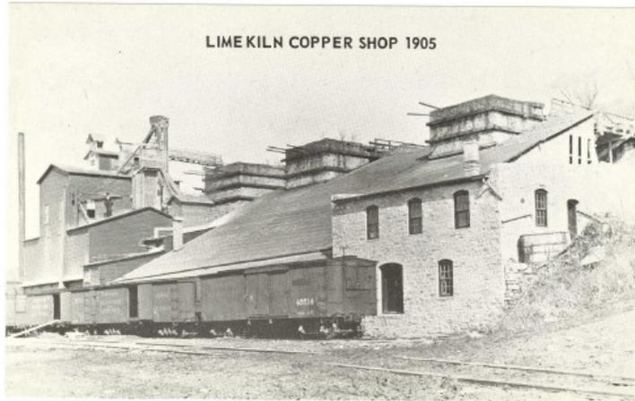
The kilns resemble tall stone ovens, and were used to “cook” limestone rocks from the sedimentary layers of limestone ledge known as the Niagara Escarpment. Chemically, limestone is largely calcium carbonate and lime is calcium oxide. Crushed limestone was heated to break down the calcium carbonate, leaving lime as the end product.
