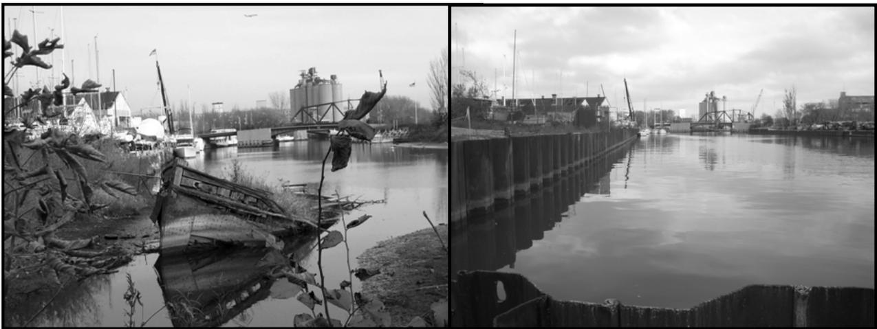
*Before and after photographs: As part of the Kinnickinnic River cleanup the project removed debris, river-choking mud flats and an abandoned boat.*
