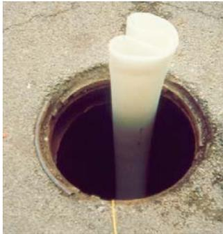
**Slip Lining:** An access pit is excavated adjacent to an existing sewer and a liner pipe of slightly smaller diameter is slid into the existing pipe to create a continuous, watertight liner between the two manholes.
