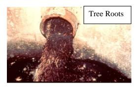
Blockages from scum, dirt, debris, grease, and roots are detected visually from digital photos. Cracks, holes, and breaks in sewer lines are also identified. Illicit discharges of cooling or heating water and other fluids can also be detected. Once these types of problems are documented, a maintenance plan to correct them can be developed.
