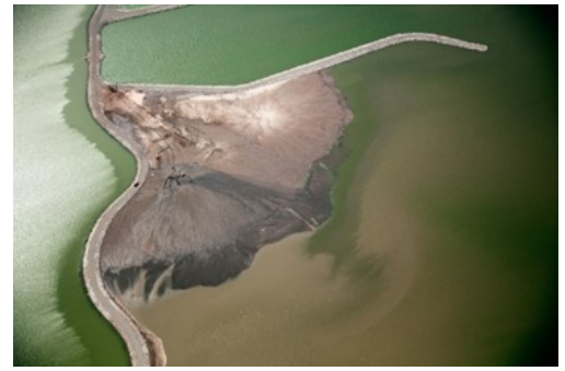
Islands take shape with clean sediment dredged from Green Bay Harbor (above) and Duluth-Superior Harbor (below). It's a cost-effective way for Great Lakes ports to maintain shipping channels.
