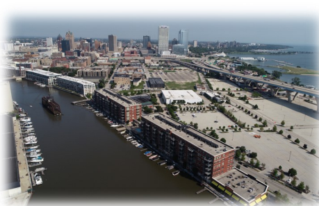
Milwaukee River at Third Ward
