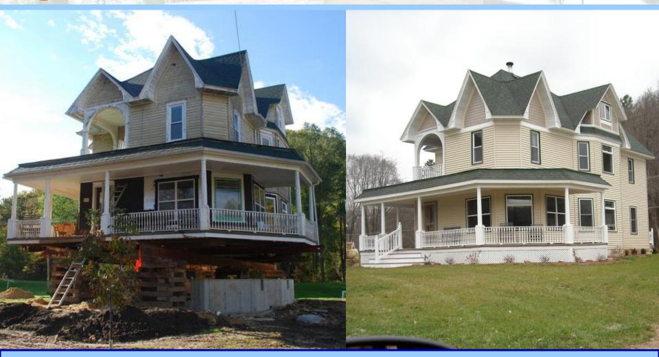
**Elevation raises a structure out of the floodplain.**
