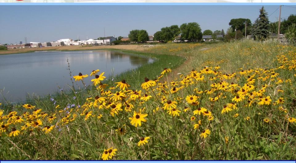
Detention/retention ponds can store storm water runoff, decreasing flash flooding in urban areas.
