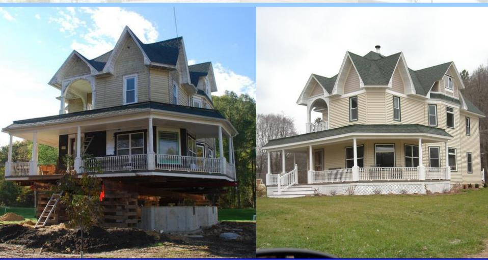
Elevation raises a structure out of the floodplain.
