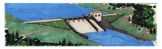
**GRAVITY DAM** - A dam constructed of concrete and/or masonry that relies on its weight for stability.
