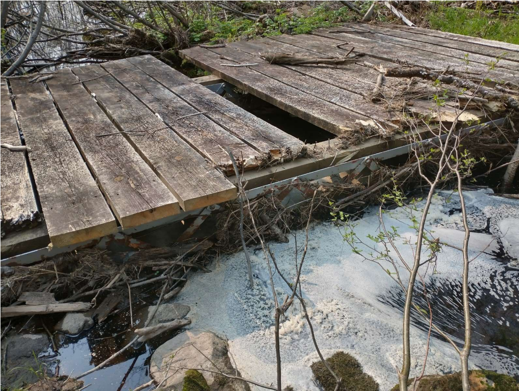
Bridge from upstream
