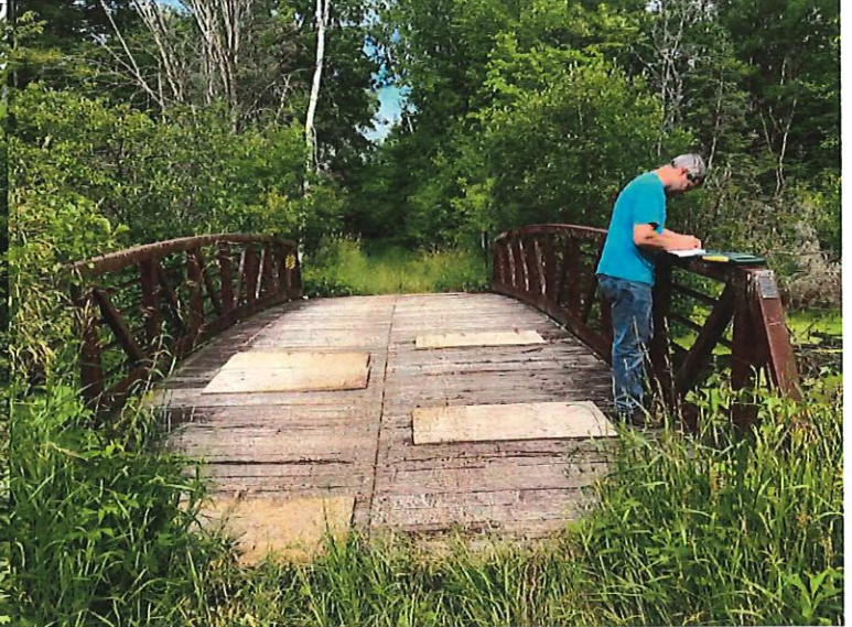
Bridge Deck Looking East
