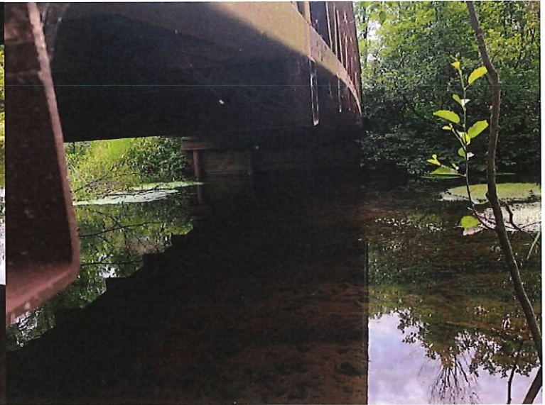
Bridge Substructure and Abutment Looking East
