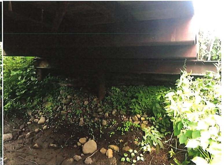
Bridge Substructure and Abutment Looking East
