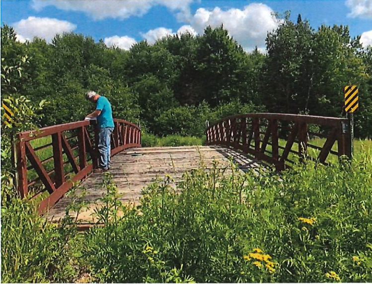
Bridge Deck Looking West
