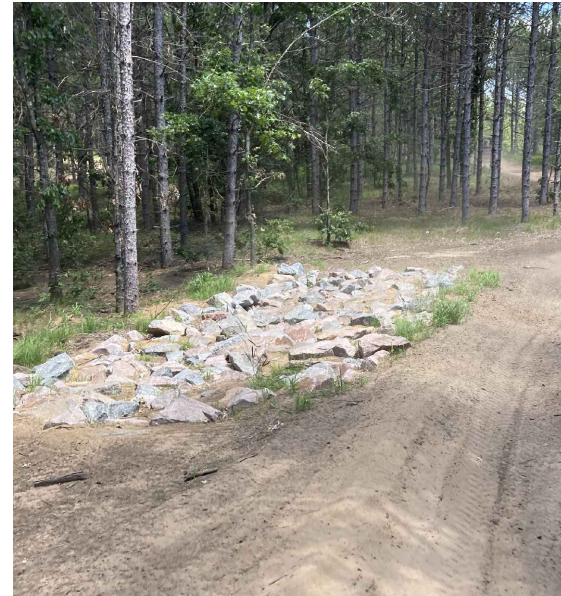
OBSTACLE 2 - MED/LARGE RIPRAP
