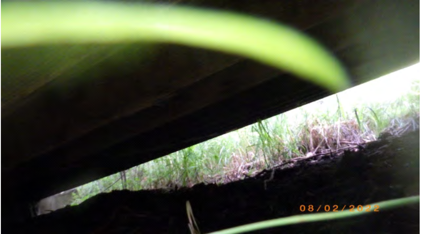
Bridge 1 (B1), Bottom of girders, end of East span.
