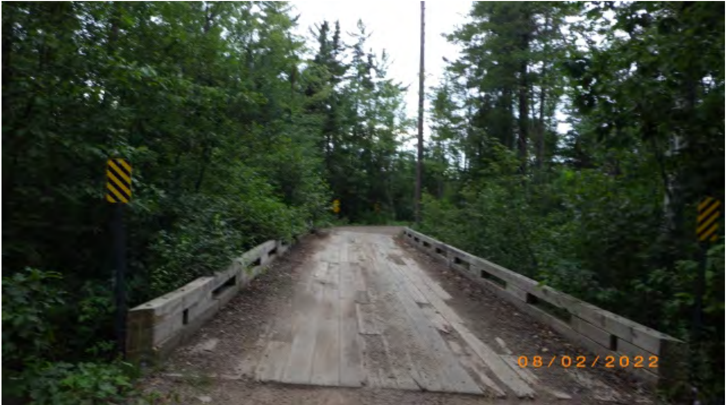
Cut brush typical of all the bridges.
