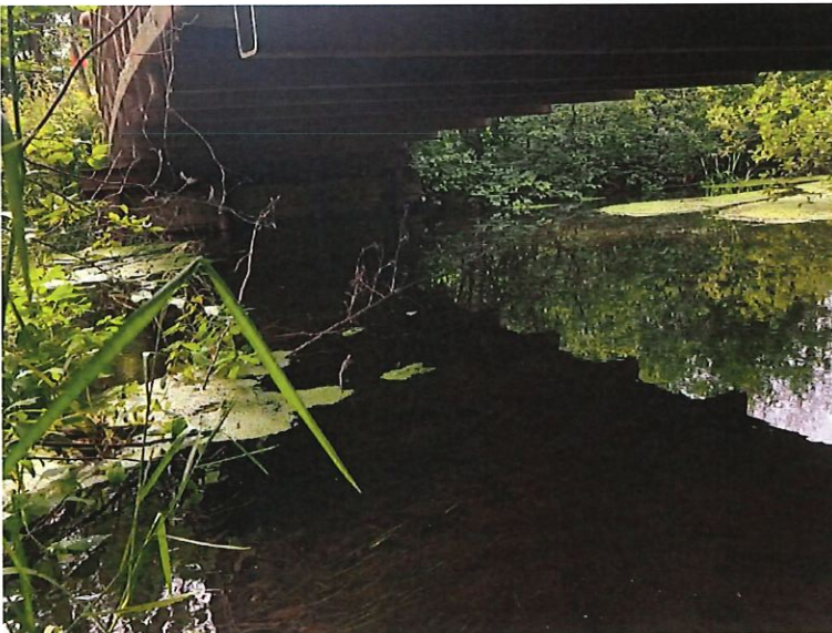
Bridge Substructure and Abutment Looking West
