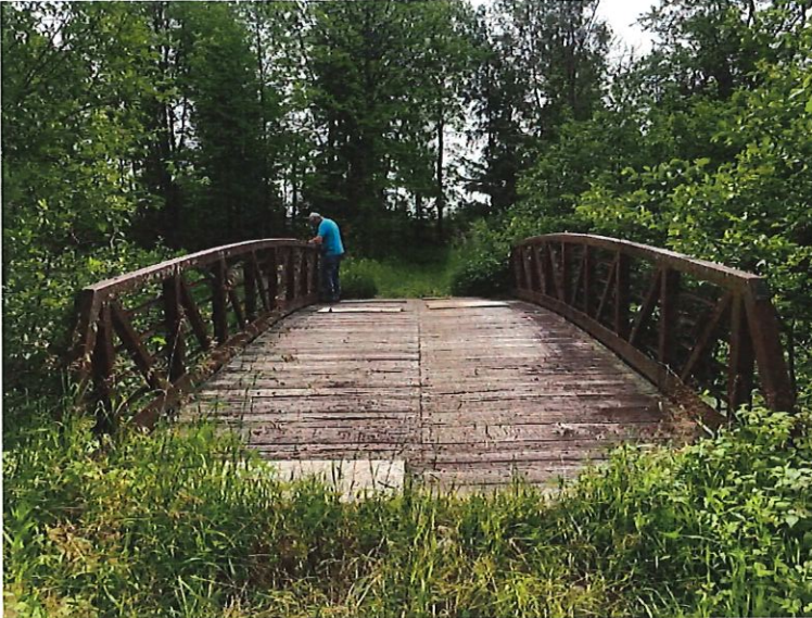
Bridge Deck Looking West
