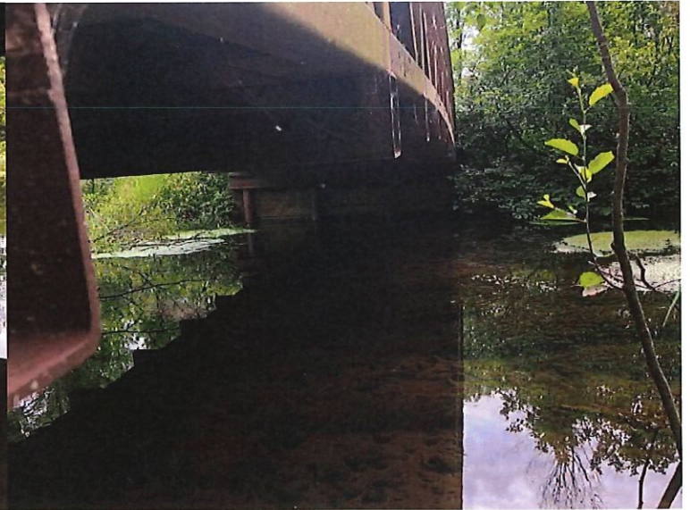
Bridge Substructure and Abutment Looking East
