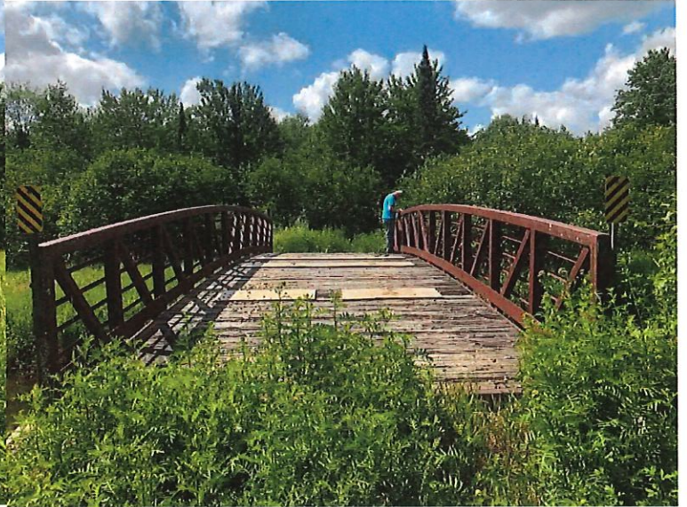
Bridge Deck Looking East
