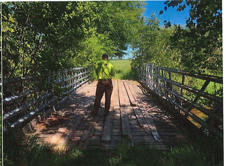
Bridge Deck Looking East
