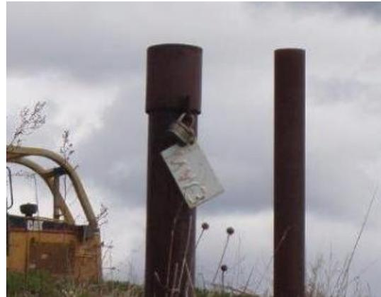
**Figure 3.** Photo of metal well label with a welding bead used to write the name of well on the label. This can be made in a shop and installed in the field without bringing a welder to the well.
