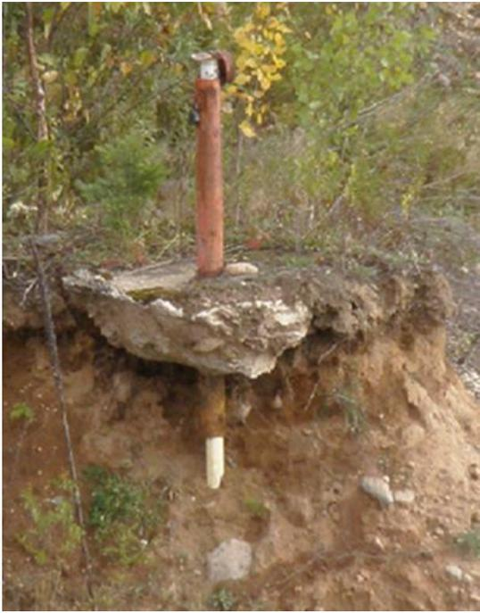
**Figure 1.** As a result of neglect, soil erosion around the cement surface seal exposed the PVC well casing. Replacing the well may be the only option.
