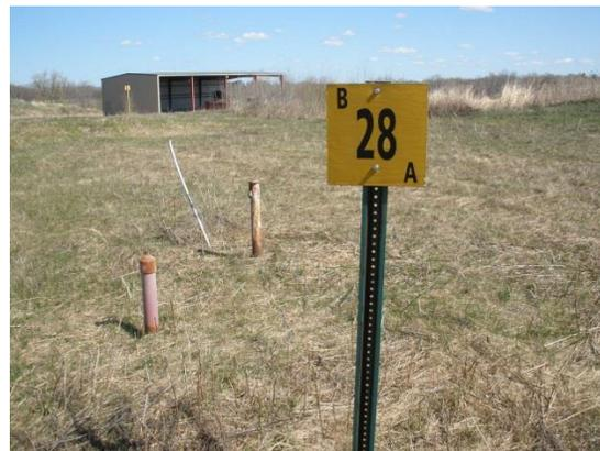
**Figure 4.** Sign with well name near the well. While the label is not on the casing, this is acceptable if it is clear which well the sign is identifying.
