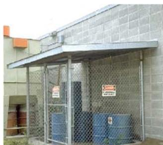
55-gallon drums are under cover and have secondary containment
