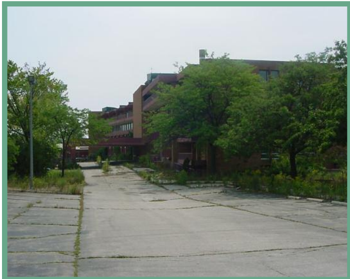
The overgrown parking lot at the site of the vacant Shores rehabilitation facility and nursing home (photo courtesy DNR).
