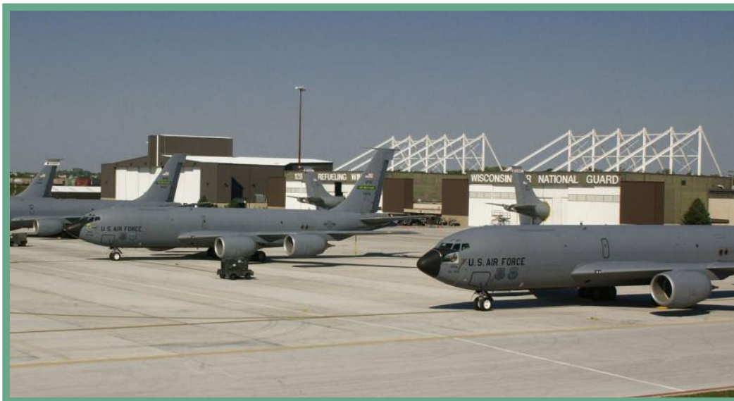
DNR staff assisted the Wisconsin Air National Guard in meeting environmental regulations while expanding the concrete apron where the aircraft are parked (photo courtesy Wisconsin Air National Guard).
