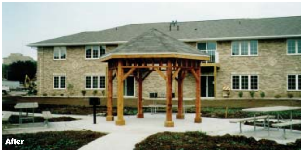
The new Radford Village is home to UW-Oshkosh students. The courtyard seen here serves as a cap to protect people from exposure to lead contamination that remains in the soil.
