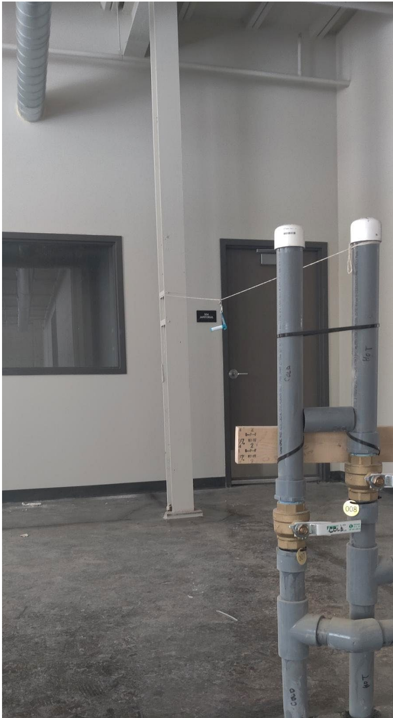
Picture 2 – Passive Sampler Location in Building 5
