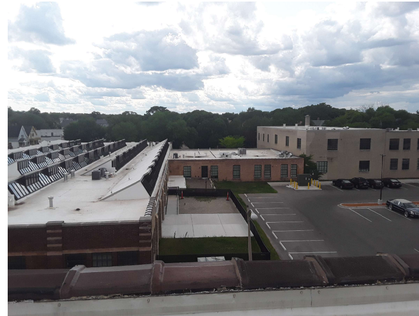
Photo taken July 17, 2023 showing Building 5 Venting Modifications
