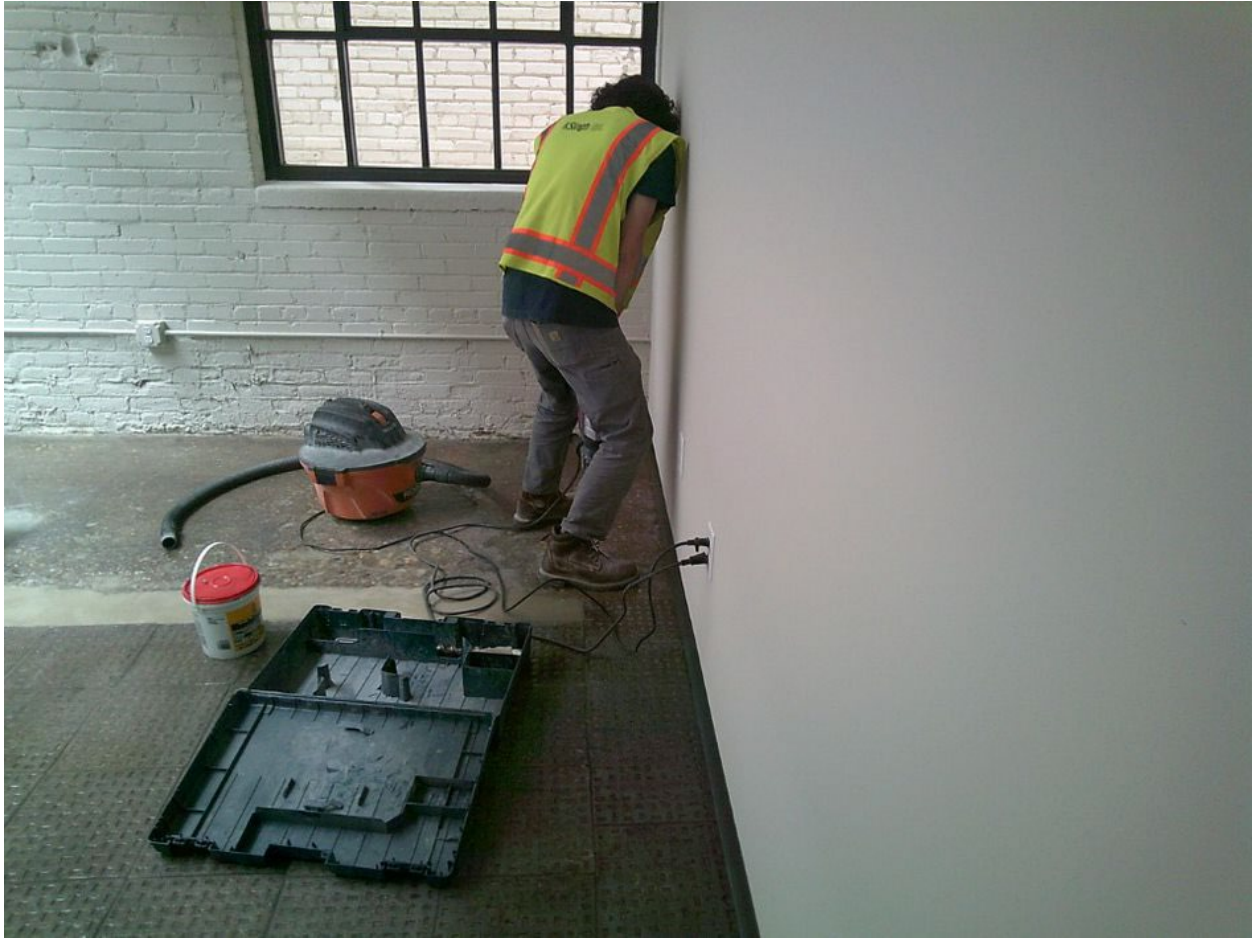
Picture 1. Vapor Pin Installation
