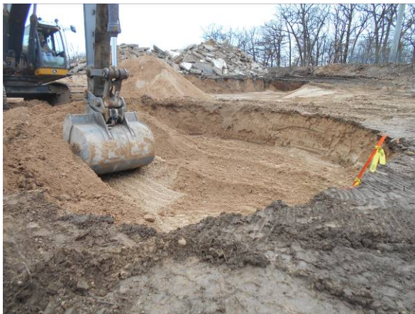
Photo #3 View looking south at B-5/B-5A excavation area.
