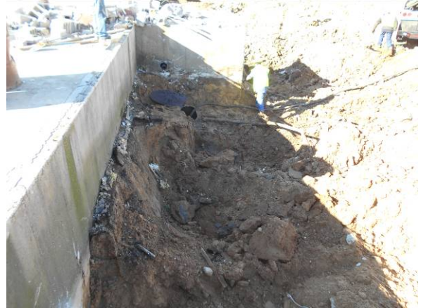
Photo #14 View looking west of east tank during liquid removal/cleaning prior to removal.
