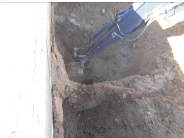
Photo #17 View looking at east tank excavation.
