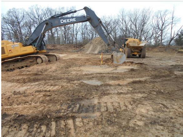
Photo #1 View looking west at B-5/B-5A area prior to excavation.
