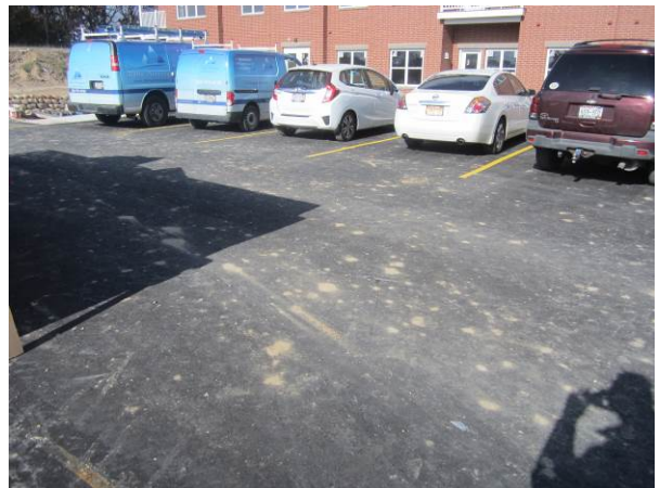
Photo #30 View north at northern cap area.
