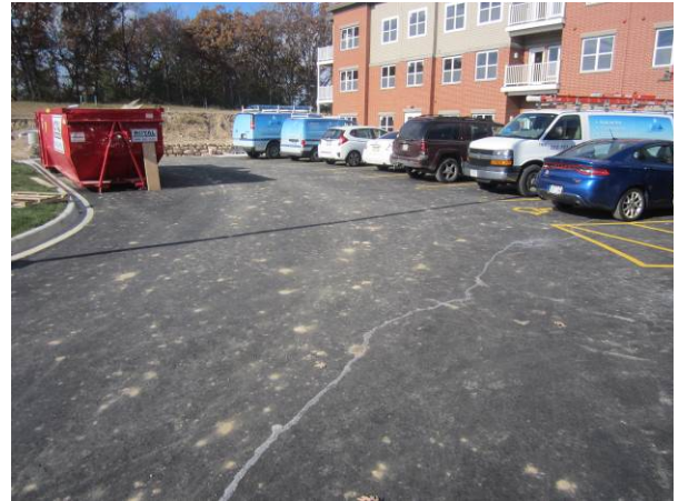
Photo #32 View looking west at northern cap area.
