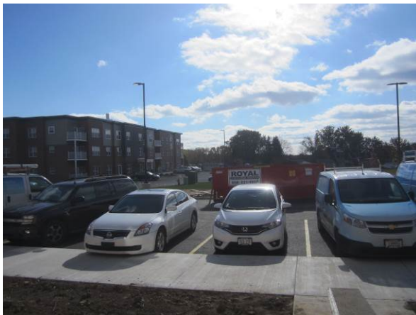
Photo #29 View looking south at northern cap area.
