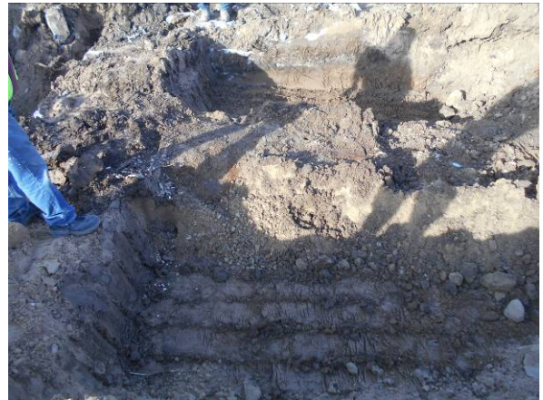
Photo #10 View of west tank prior to removal.
