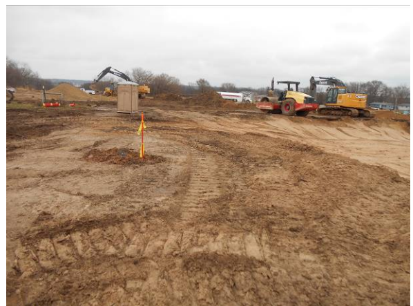
Photo #6 View looking east at B-10 excavation area prior to excavation
