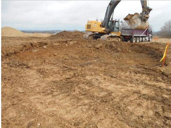
Photo #7 View looking north east at B-10 excavation area during excavation.
