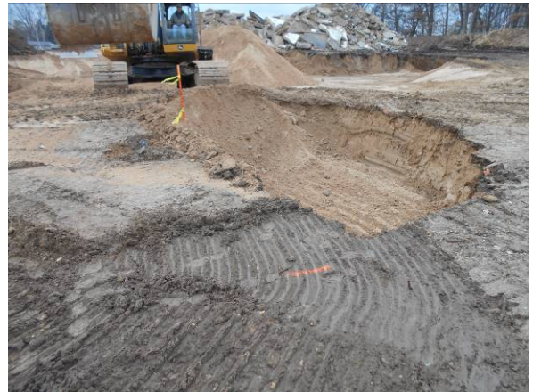
Photo #2 View looking south at B-5/B-5A excavation area.
