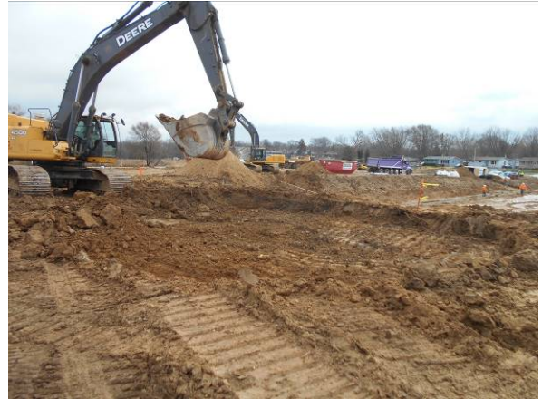
Photo #8 View looking east at B-10 excavation area during excavation.
