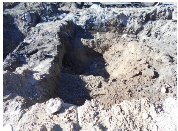
Photo #12 View of west tank excavation after west tank removed.
