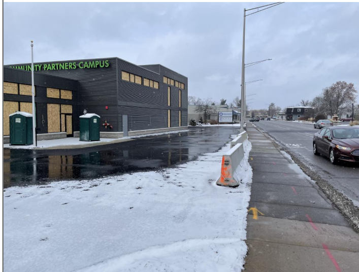
Title: View north-northwest along eastern property boundary.
