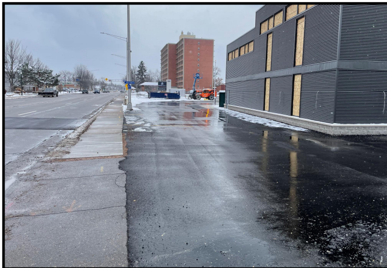
View south-southeast along eastern property boundary.
