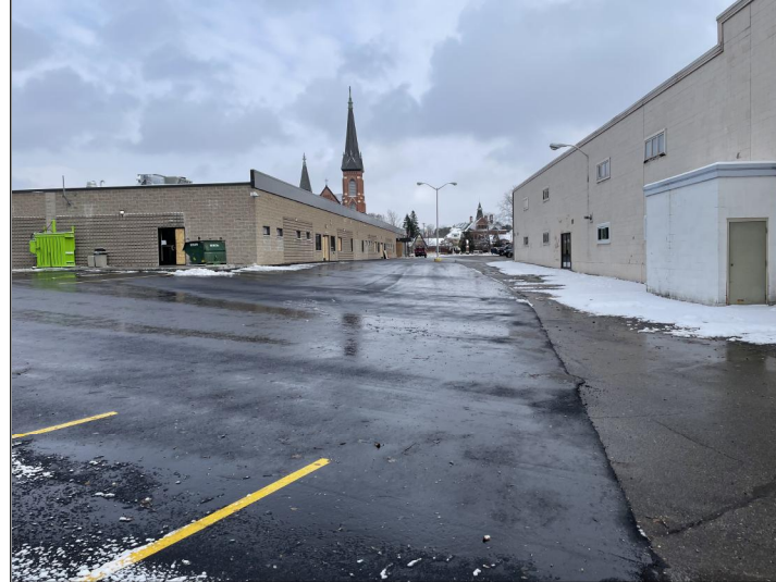
Title: View north-northeast along western property boundary.
