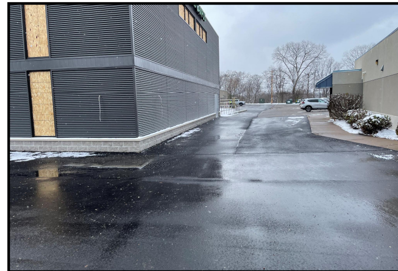
View west-southwest along northern property boundary.
