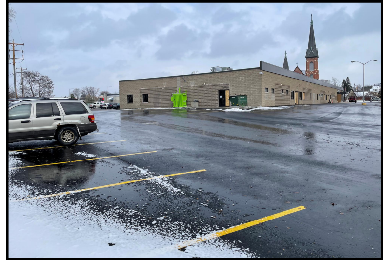
View northeast towards site structure.
