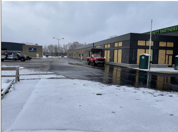
Title: View west-southwest along southern property boundary.
