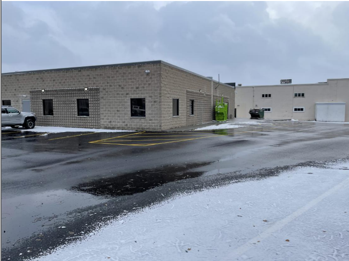
Title: View southwest towards site structure.
