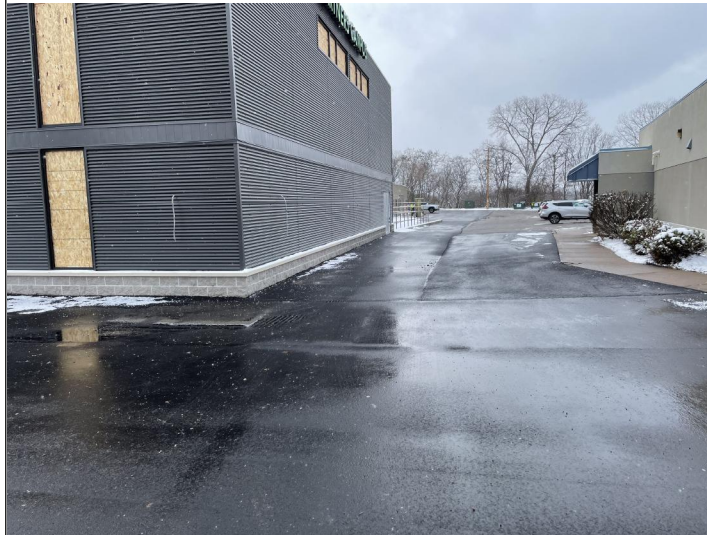
Title: View west-southwest along northern property boundary.
