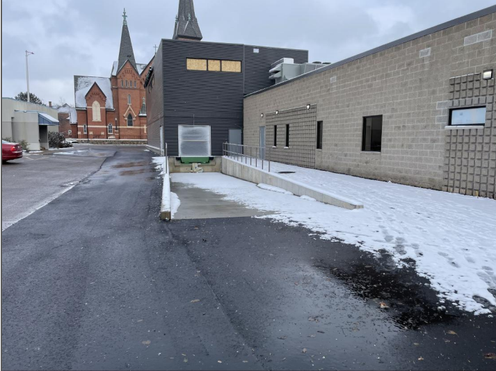
Title: View east towards loading dock.
