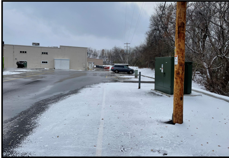
View northeast towards site structure.
