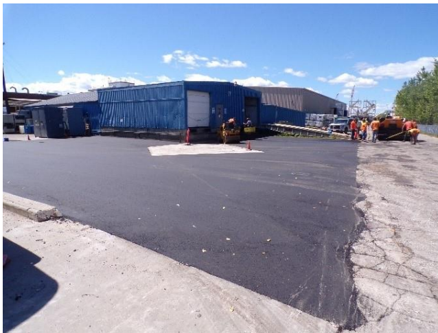
Photograph 1: Cover Area D Asphalt Replacement
