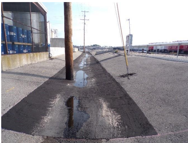
Photograph 2: Cover Area H Asphalt Repair
