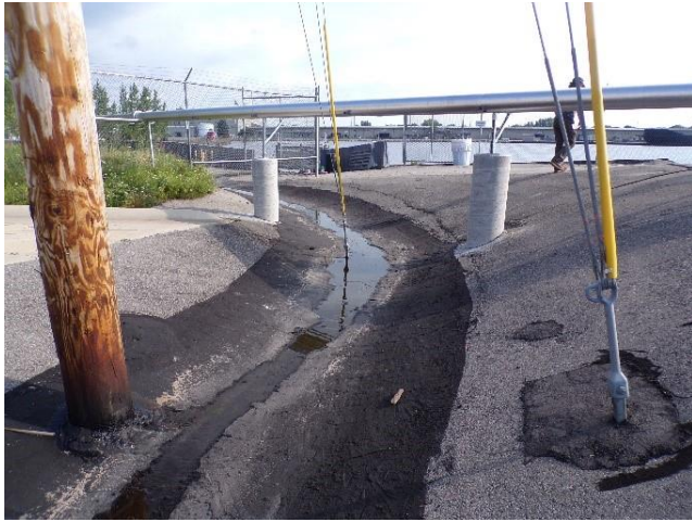
Photograph 3: Cover Area H Asphalt Repair
