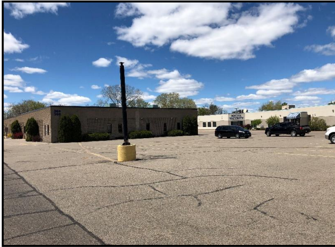
View northwest toward on-site structure.
