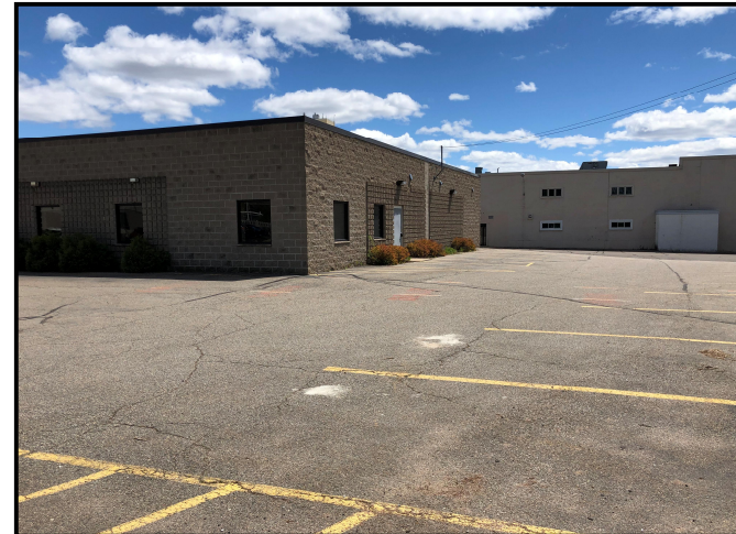
View southeast toward on-site structure.
