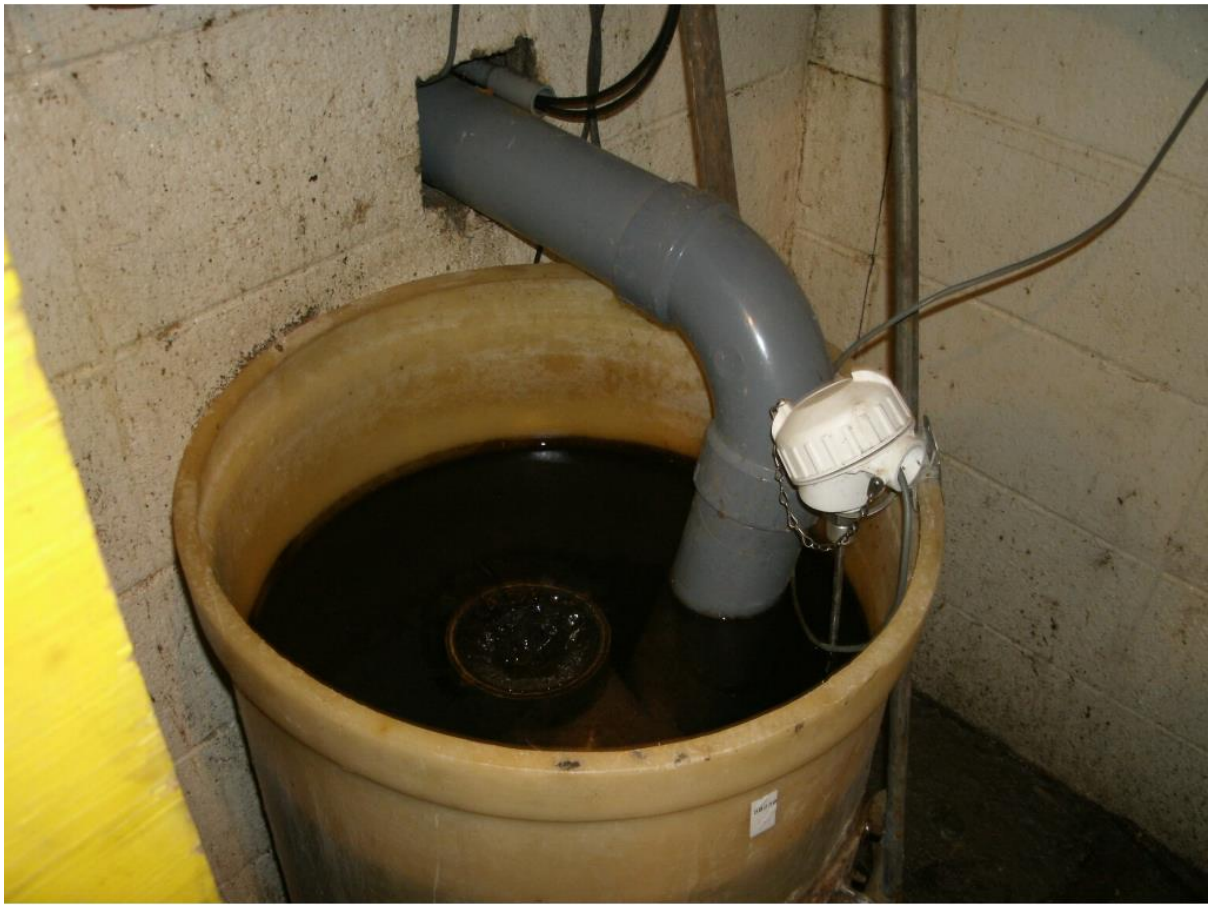
Sampling Location for Outfall 001
