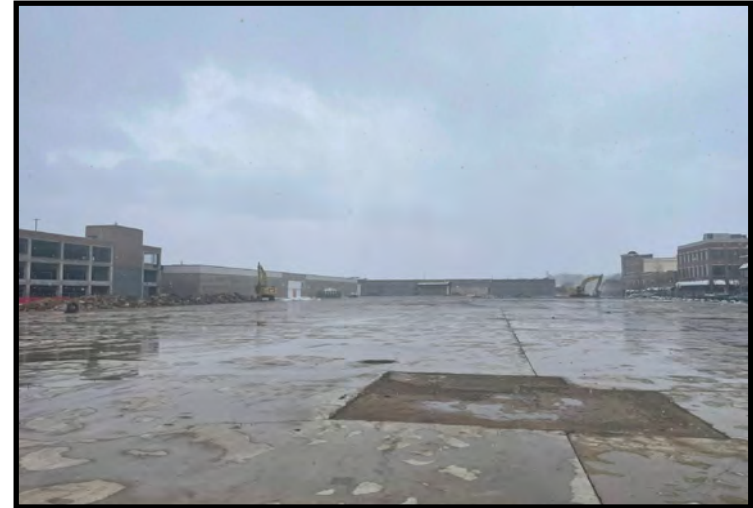
Removal of concrete cap (04/18/2023)
