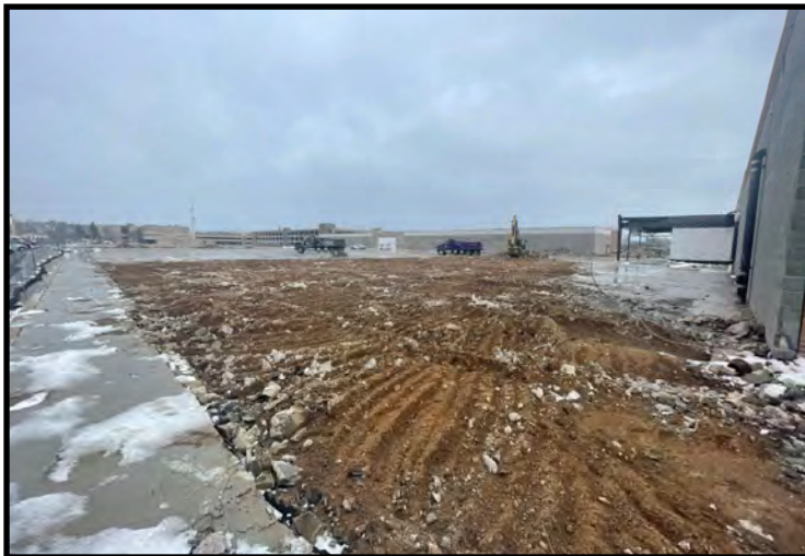
Removal of concrete cap along 2nd Street (04/19/2023)
