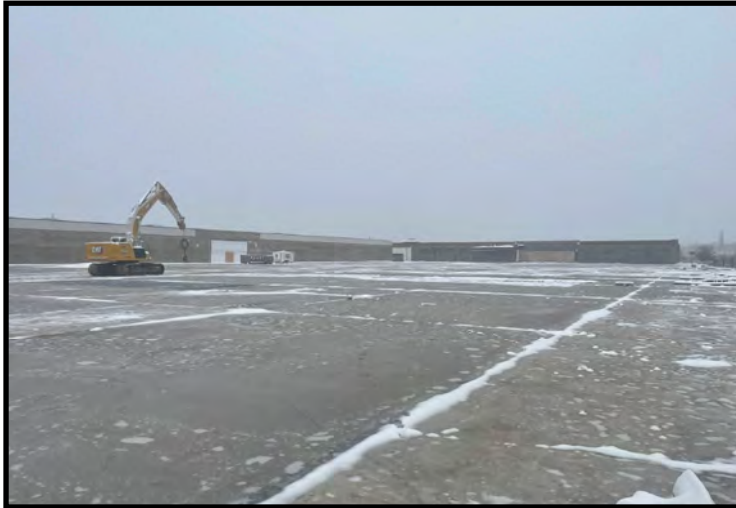
Intact concrete cap prior to redevelopment work (04/17/2023)
