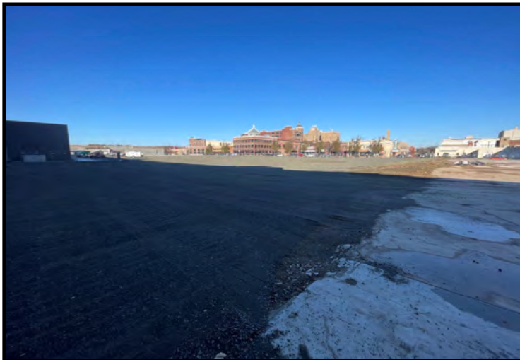
Temporary gravel cap over Block 4 and 3rd Street (11/09/2023)
