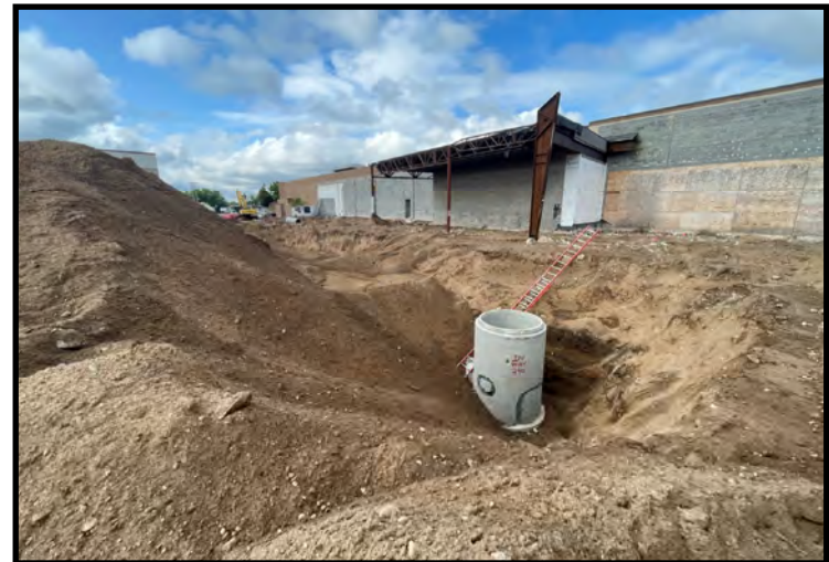
Utility installation within 2nd Street right-of-way (09/11/2023)
