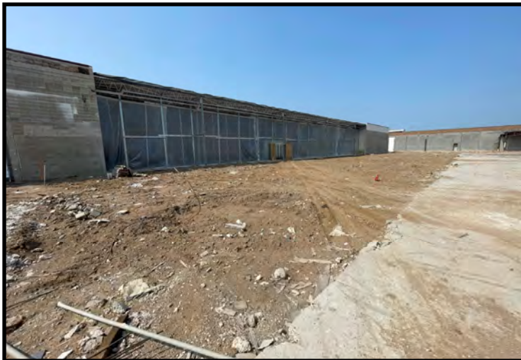
Uncapped area north of HOM Furniture prior to redevelopment (06/16/2023)
