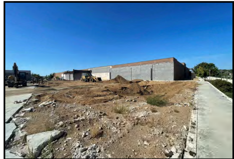
Excavation of northern portion of 2nd Street right-of-way (09/01/2023)
