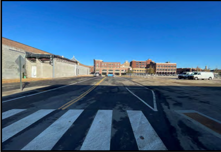
Asphalt cap over 2nd Street right-of-way (11/09/2023)
