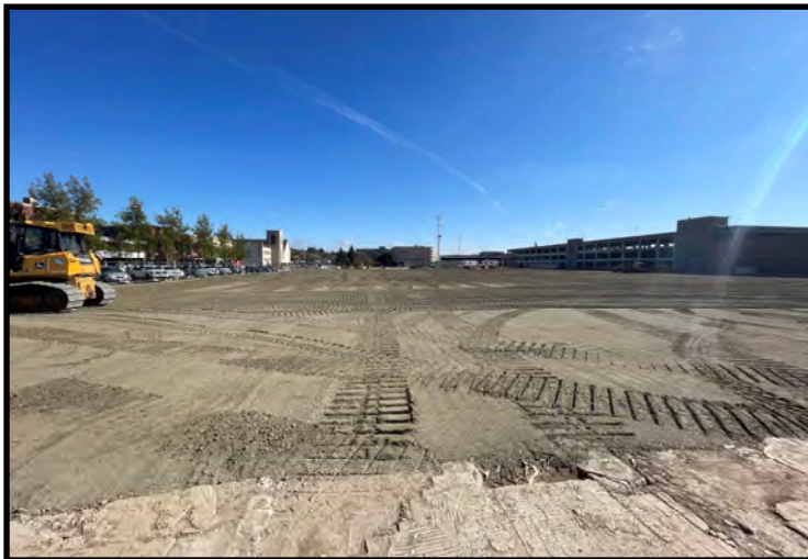
Temporary gravel cap over Block 4 and 3rd Street (10/17/2023)
