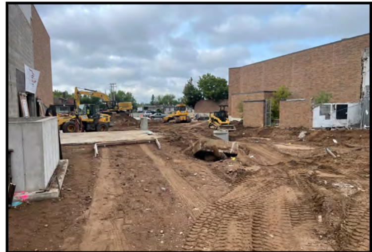
Utility installation within 2nd Street right-of-way (08/29/2023)
