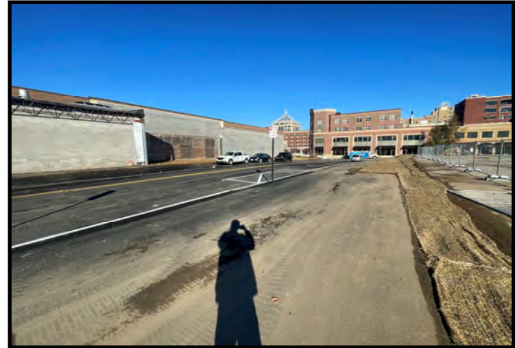
Asphalt cap over 2nd Street right-of-way (11/09/2023)
