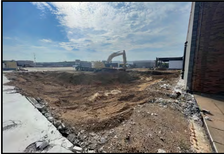
Excavation of northern portion of 2nd Street right-of-way (09/05/2023)
