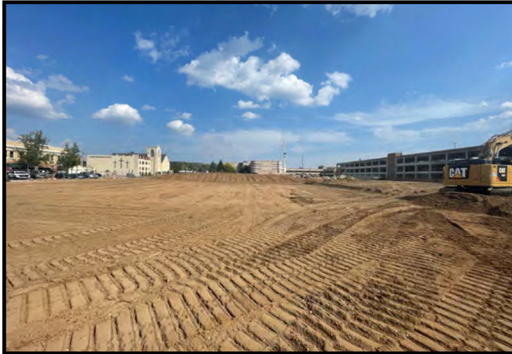
Reg grading of Block 4 (09/21/2023)
