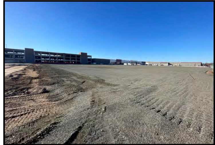
Temporary gravel cap over Block 4 and 3rd Street (11/09/2023)
