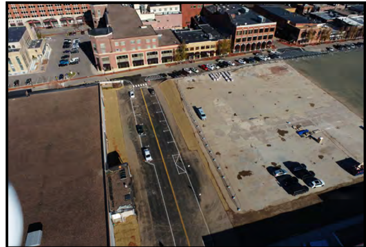
Drone photo depicting current conditions (11/13/2023)
