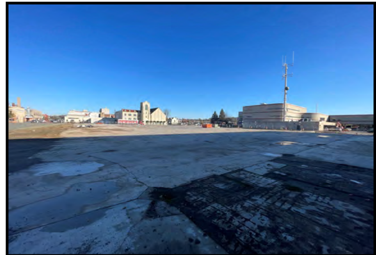
Concrete cap over Block 5 (11/09/2023)
