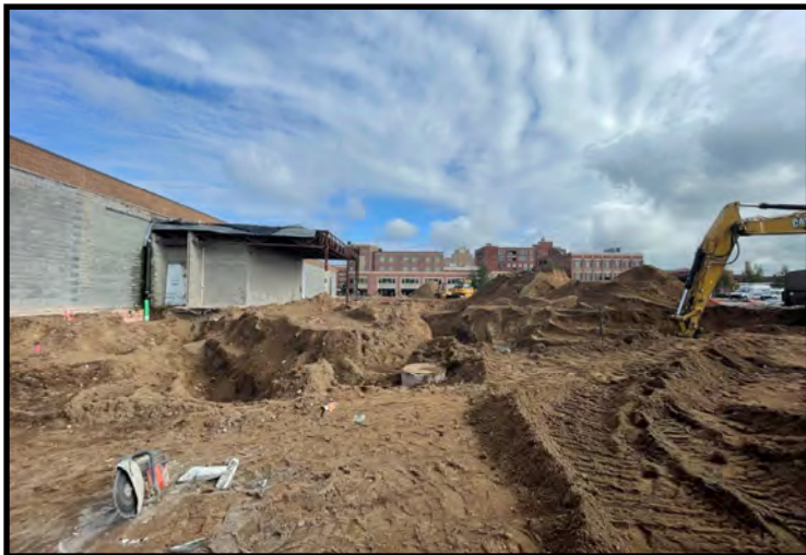
Utility installation within 2nd Street right-of-way (09/11/2023)
