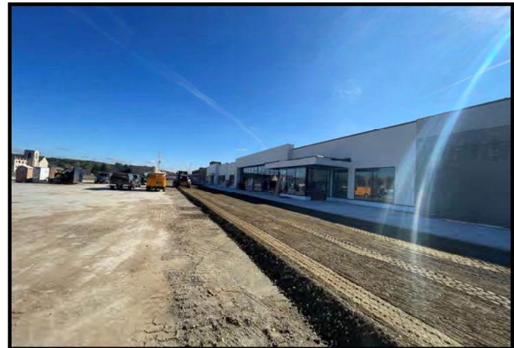
Reg grading of area in front of HOM Furniture (10/17/2023)
