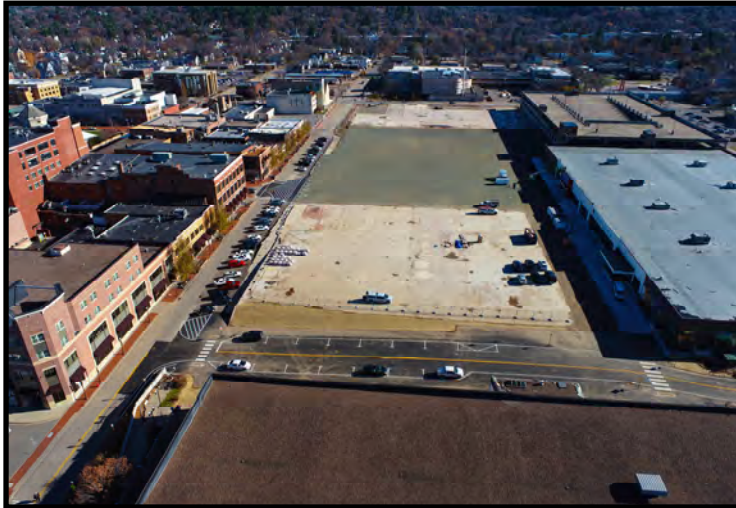
Drone photo depicting current conditions (11/13/2023)
