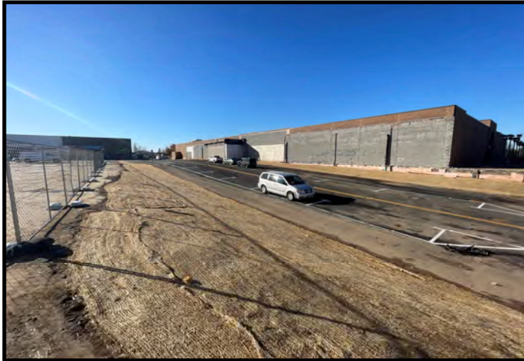
Asphalt cap over 2nd Street right-of-way (11/09/2023)
