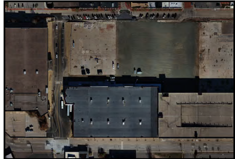
Drone photo depicting current conditions (11/13/2023)
