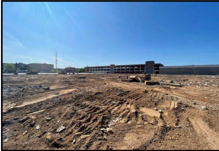
Uncapped Block 4 area prior to redevelopment (05/26/2023)
