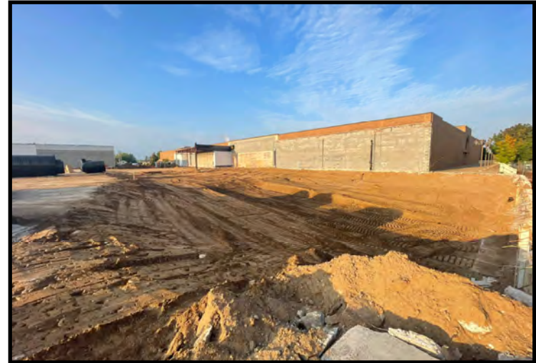
Reg grading of 2nd Street (09/21/2023)
