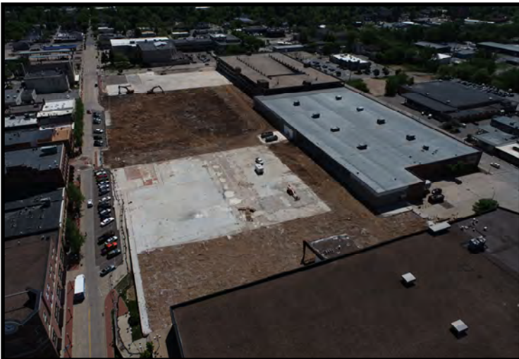
Drone photo depicting cap removal (05/25/2023)
