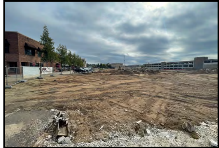
Regrading of Block 4 (09/19/2023)
