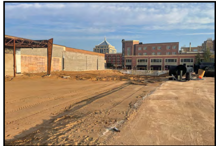
Regrading of 2nd Street (09/21/2023)
