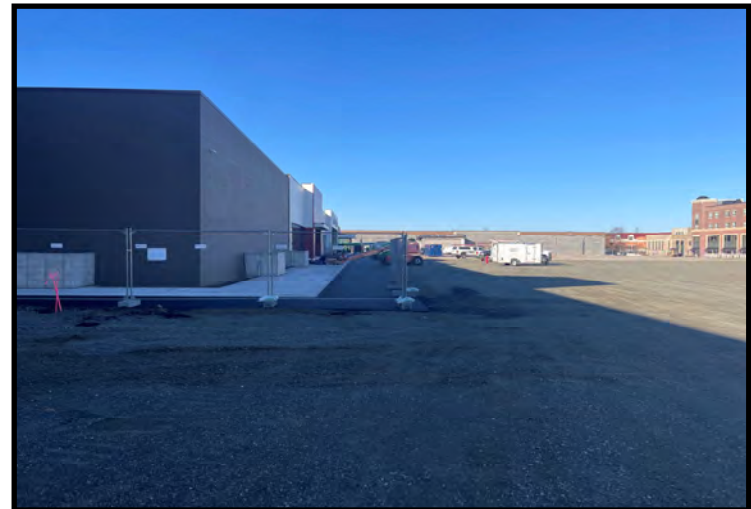
Concrete/asphalt/gravel cap over area in front of HOM Furniture building (11/09/2023)
