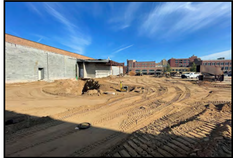
Regrading of central portion of 2nd Street (09/01/2023)
