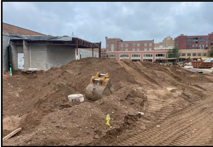
Utility installation within 2nd Street right-of-way (08/29/2023)
