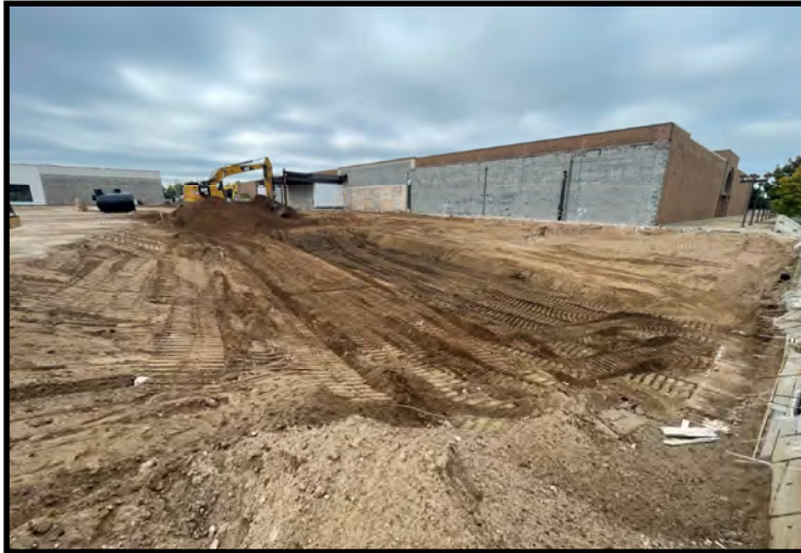
Excavation of northern portion of 2nd Street right-of-way (09/19/2023)
