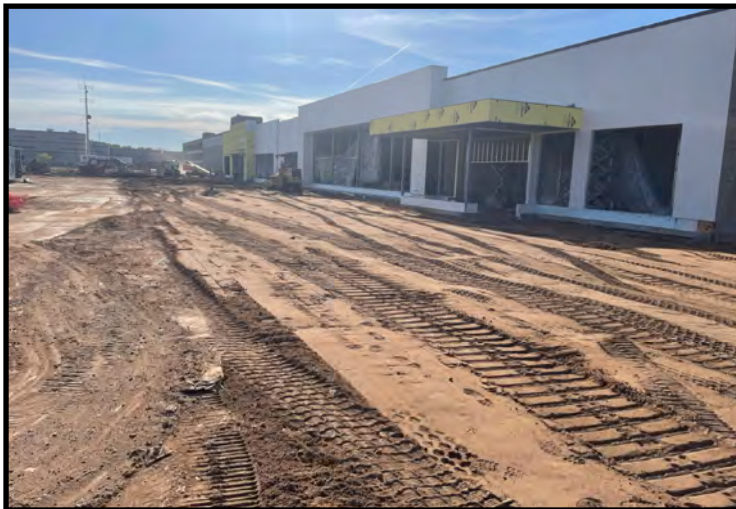
Regrading of area north of HOM Furniture (09/01/2023)
