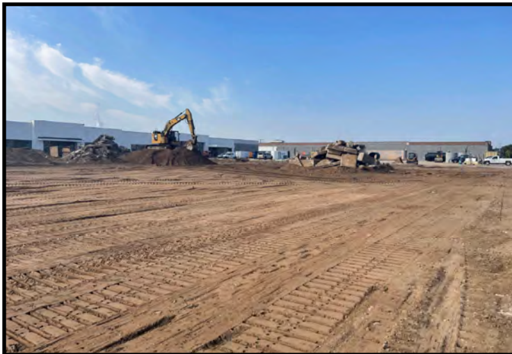
Regrading of Block 4 (09/21/2023)
