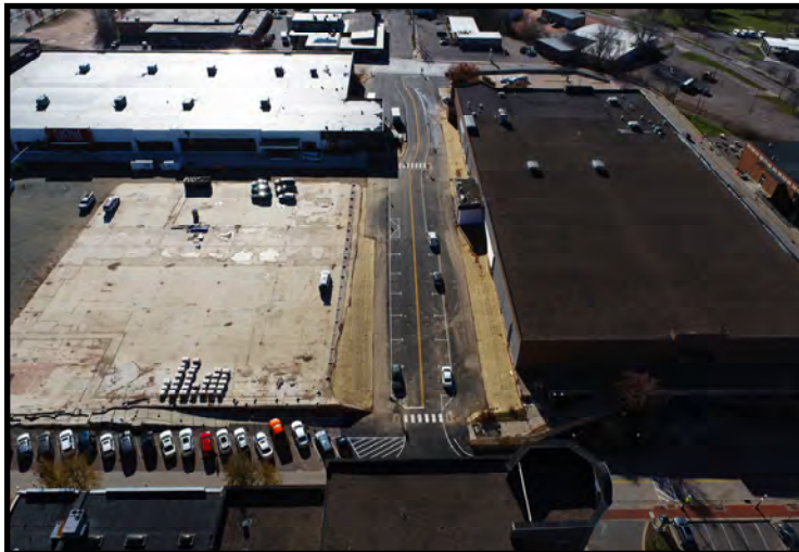
Drone photo depicting current conditions (11/13/2023)
