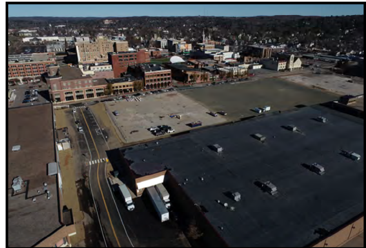
Drone photo depicting current conditions (11/13/2023)
