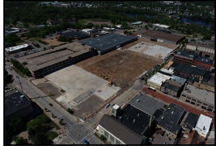
Drone photo depicting cap removal (05/25/2023)
