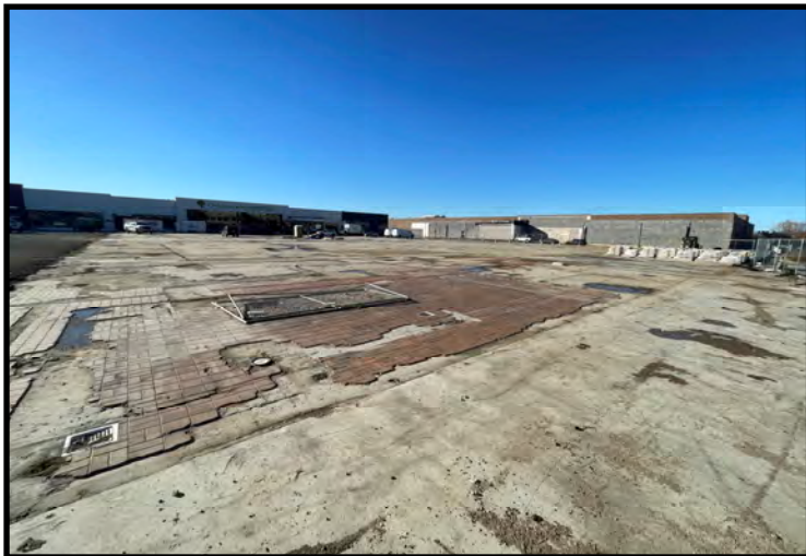
Concrete cap over Block 3 (11/09/2023)
