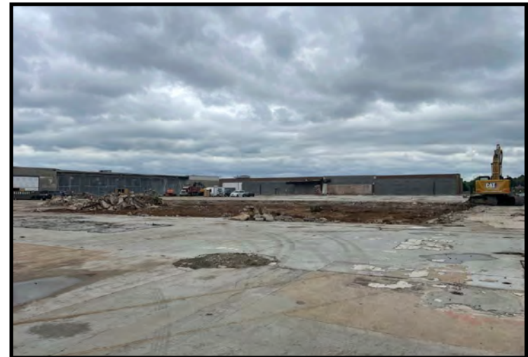
Removal of concrete cap along 3rd Street (04/20/2023)
