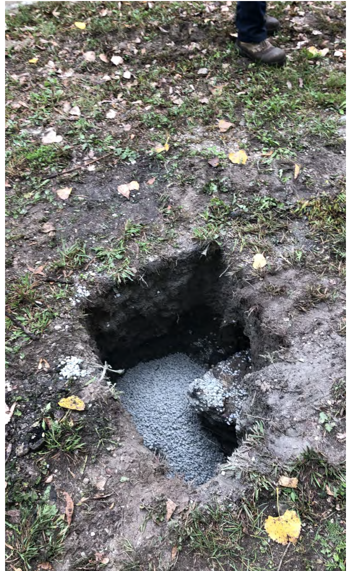
Photo 4: Geoprobe boring (MH-1-BF) northeast of manhole MH-1 backfilled with bentonite chips. View to northeast; photograph taken on September 20, 2021.
