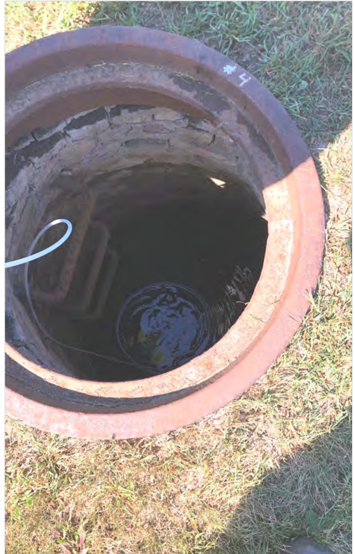
Photo 7: Manhole MH-4 interior with black & turbid water. View to north; photograph taken on September 1, 2021.
