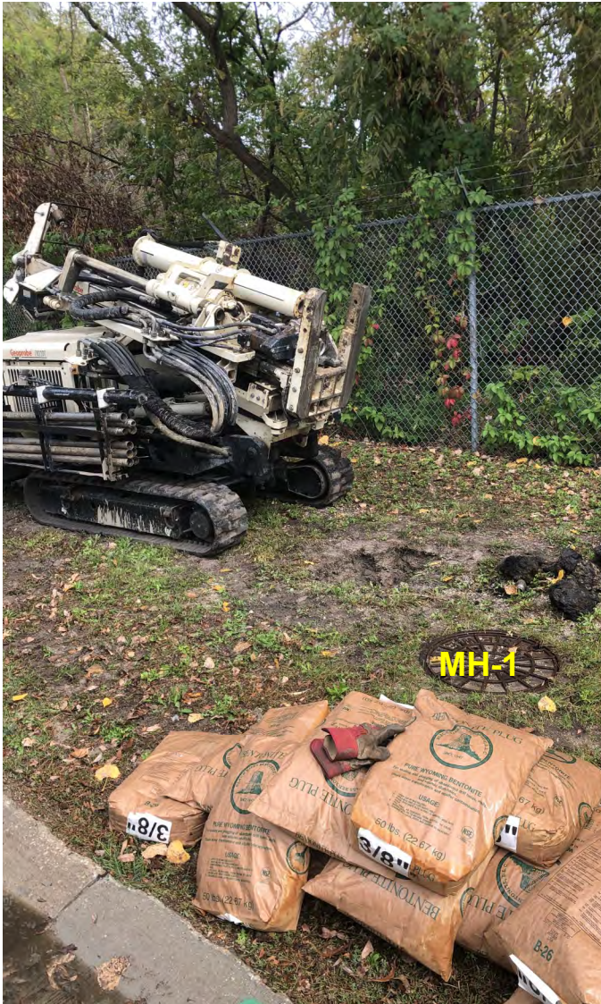
Photo 3: Geoprobe boring (MH-1-BF) within open Hydro-vac borehole northeast of manhole MH-1. View to northeast; photograph taken on September 20, 2021.
