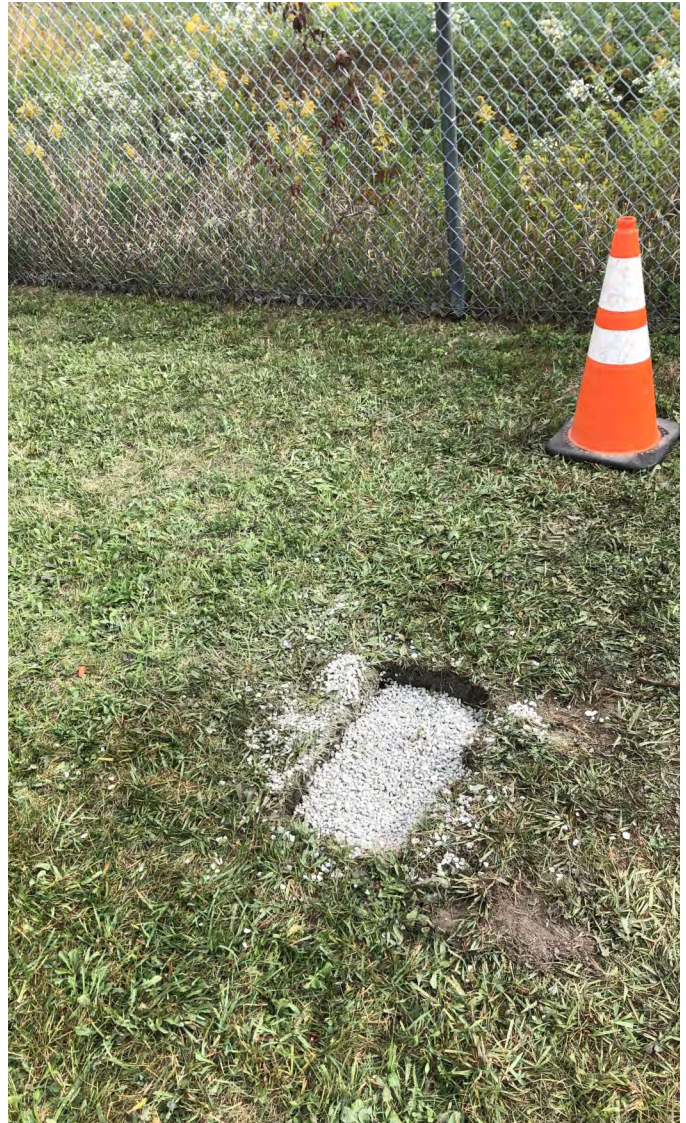
Photo 14: Geoprobe boring (MH-3-BF) northeast of manhole MH-3 backfilled with bentonite chips. View to west; photograph taken on September 20, 2021.
