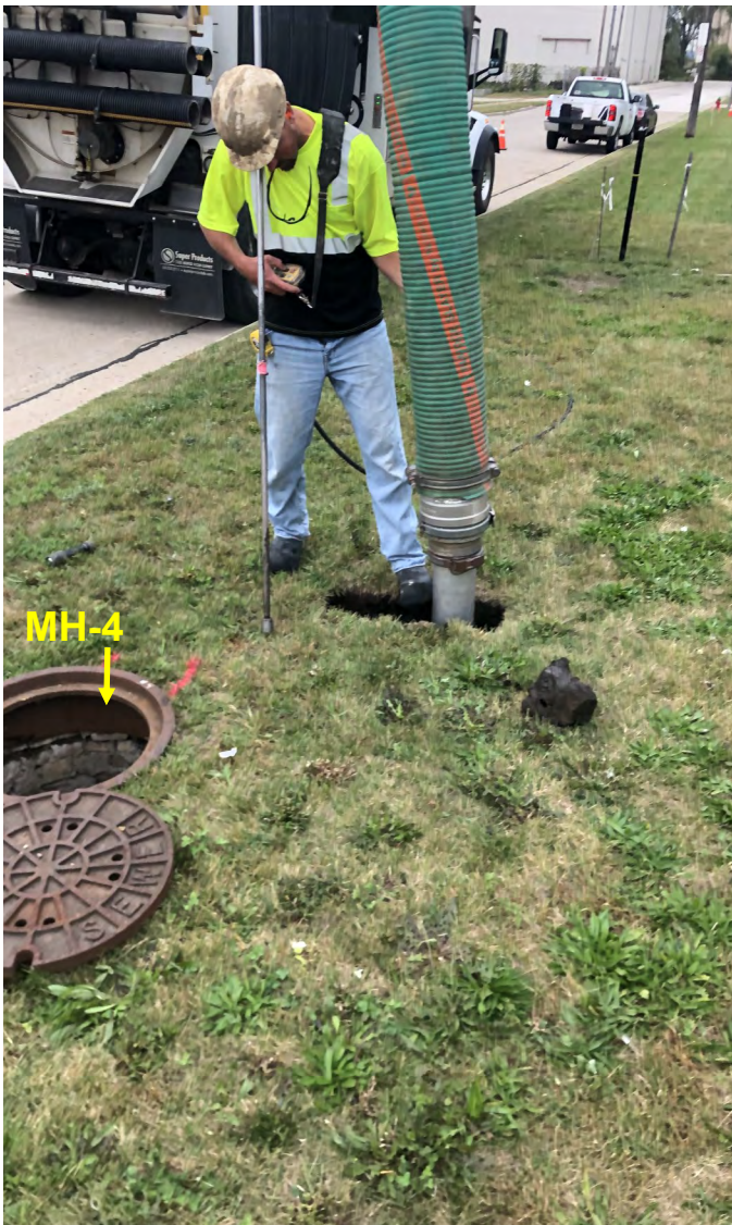
Photo 15: XPose (hydrovac contractor) conducting hydrovac excavation to the northeast of manhole MH-4. View to north; photograph taken on September 20, 2021.
