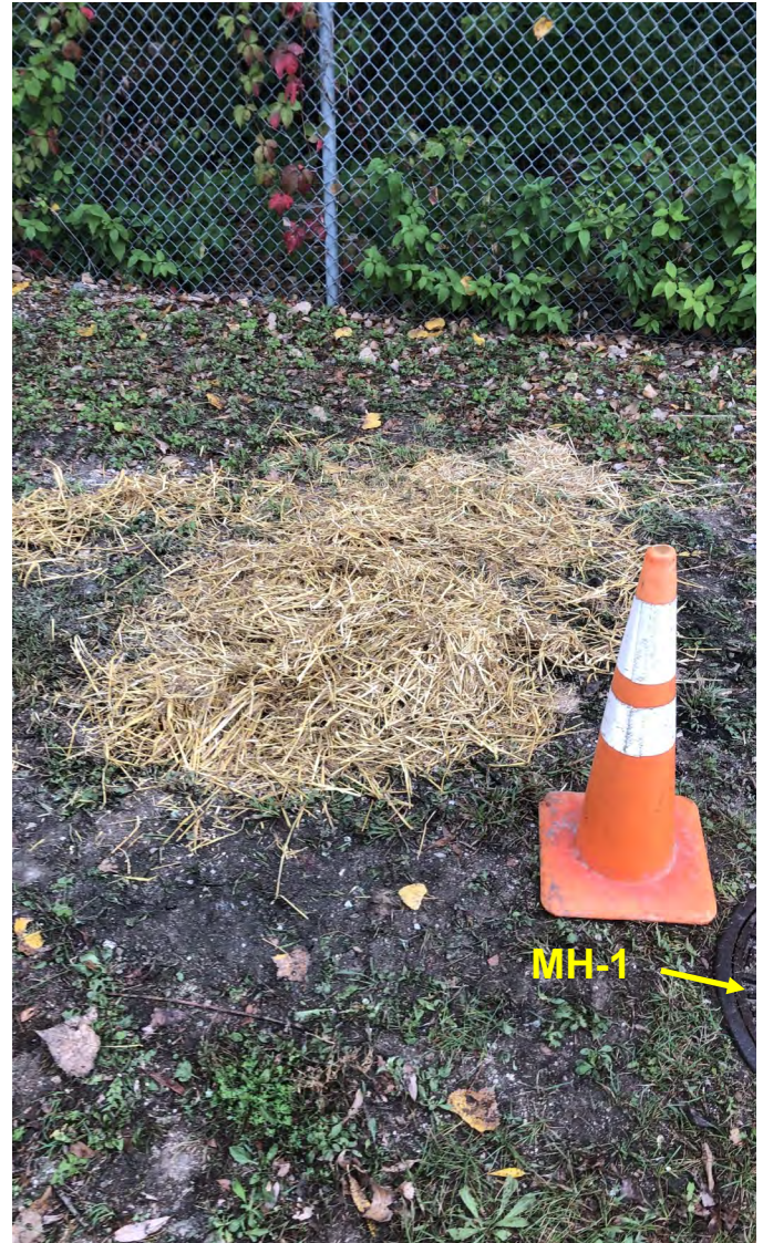
Photo 6: Geoprobe boring (MH-1-BF) borehole northeast of manhole MH-1 resurfaced with seed. View to east; photograph taken on September 20, 2021
