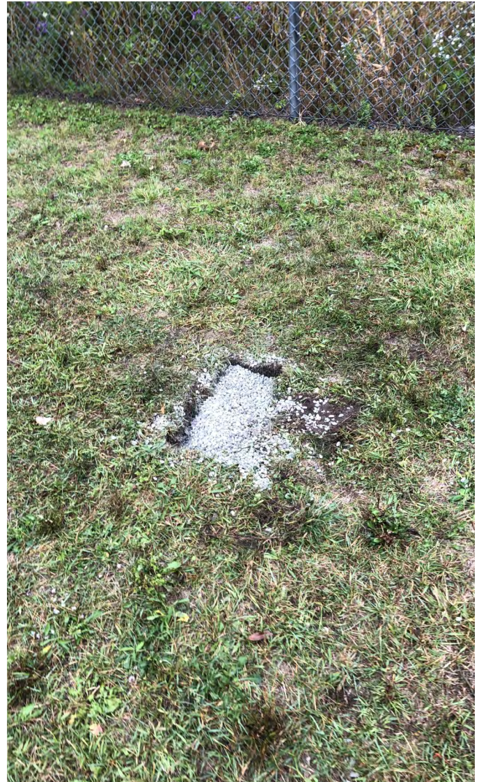
Photo 10: Geoprobe boring (MH-2-BF) northeast of manhole MH-2 backfilled with bentonite chips. View to east; photograph taken on September 20, 2021.
