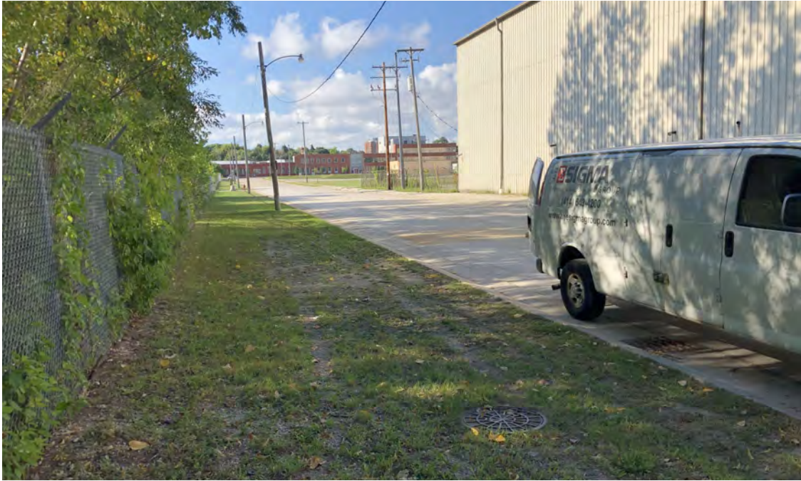
Photo 1: Manhole MH-1 within grass east of South Marina Drive. View to south; photograph taken on September 1, 2021.
