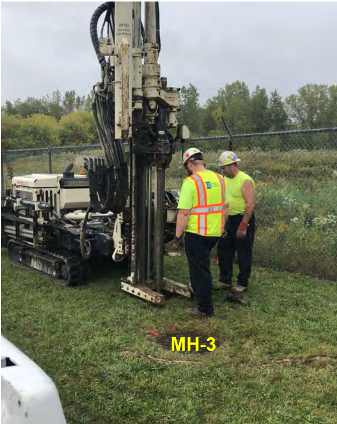
Photo 13: Geoprobe boring (MH-3-BF) within open Hydrovac borehole northeast of manhole MH-3. View to east; photograph taken on September 20, 2021.
