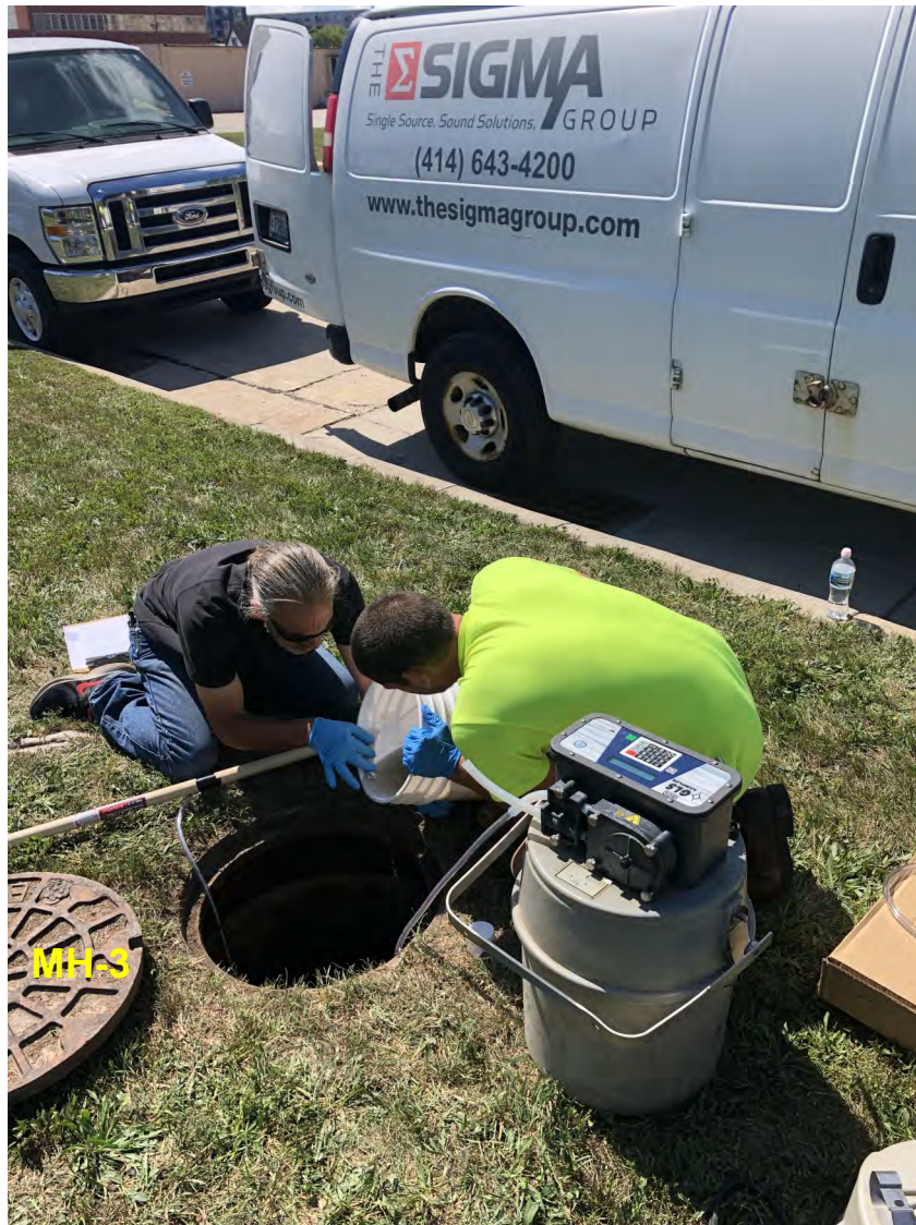
Photo 5: Manhole MH-3 within grass east of South Marina Drive. Sigma personnel decanting water from bucket. View to southwest; photograph taken on September 1, 2021.
