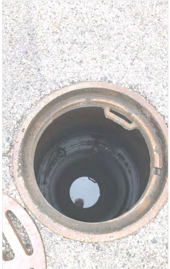
Photo 25: Manhole MH-11 interior. View to north; photograph taken on April 4, 2022,
