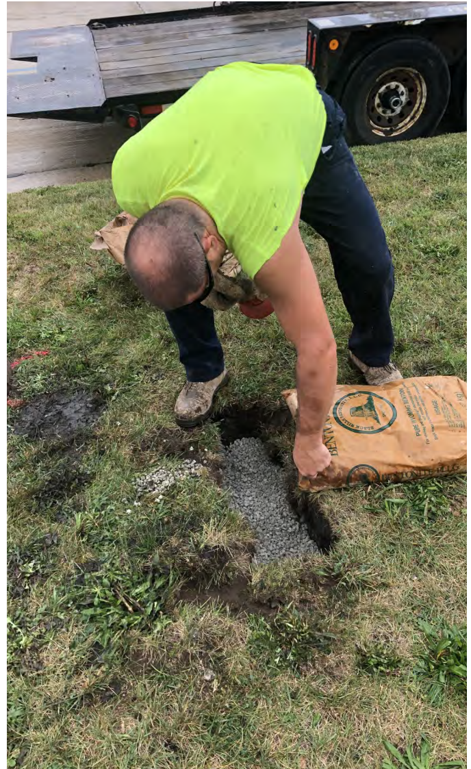
Photo 18: Geoprobe boring (MH-4-BF) northeast of manhole MH-4 backfilled with bentonite chips. View to west; photograph taken on September 20, 2021.
