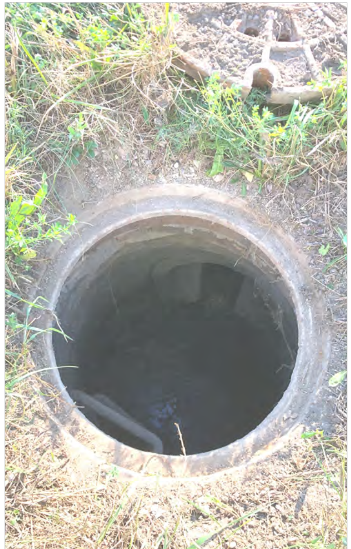
Photo 9: Manhole MH-5 interior with black & turbid water, low water column, and small amounts of sediments on bottom of SE invert. View to east; photograph taken on September 2, 2021.
