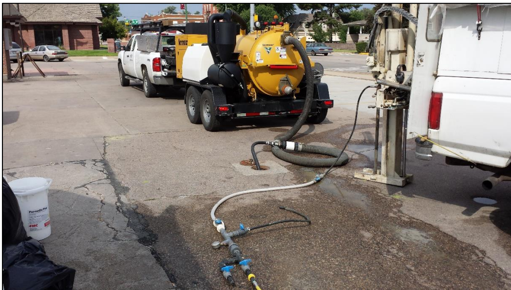
Figure 8 Vacuum extraction and in-situ injection.
