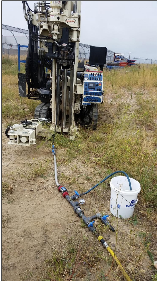
Figure 6 DPT Direct Push Technology in-situ injection.
