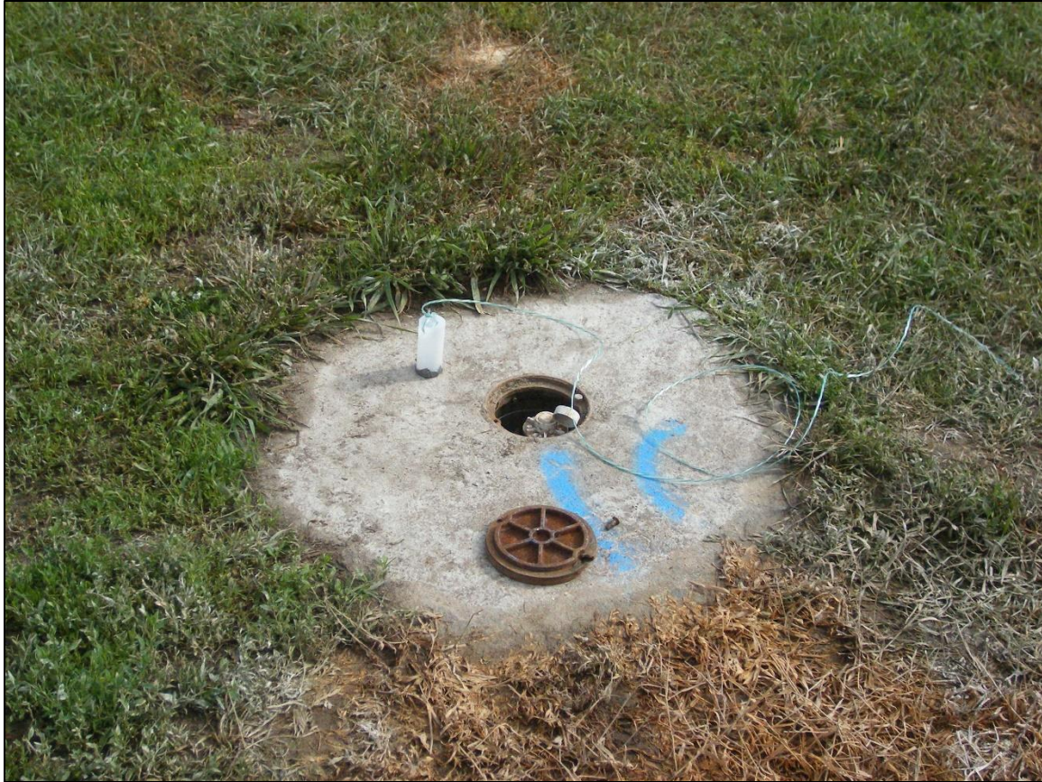
Figure 2 Flush mount monitoring well.
