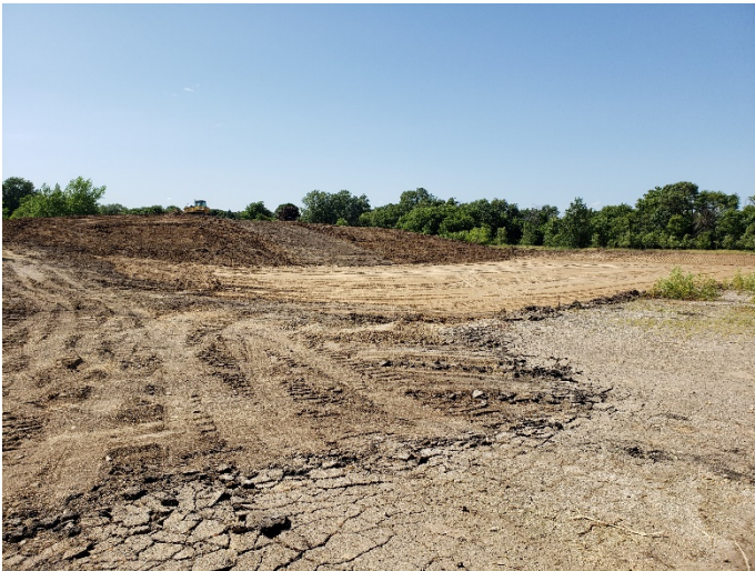
Former GM Haul Away Yard (JATCO) site receiving fill
