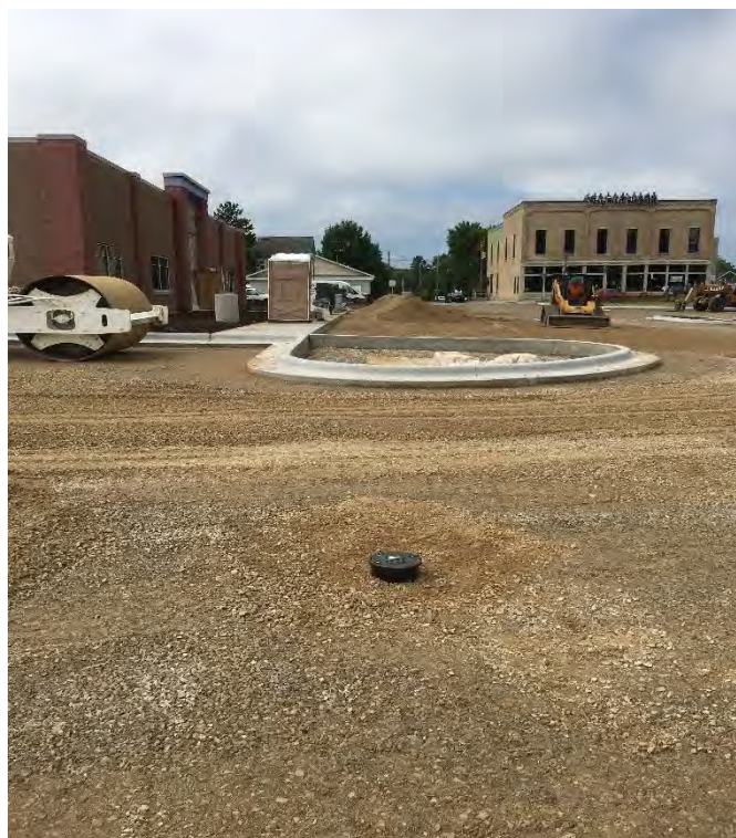
Photo 18 - Placement of gravel subgrade in parking lot; looking southwest
