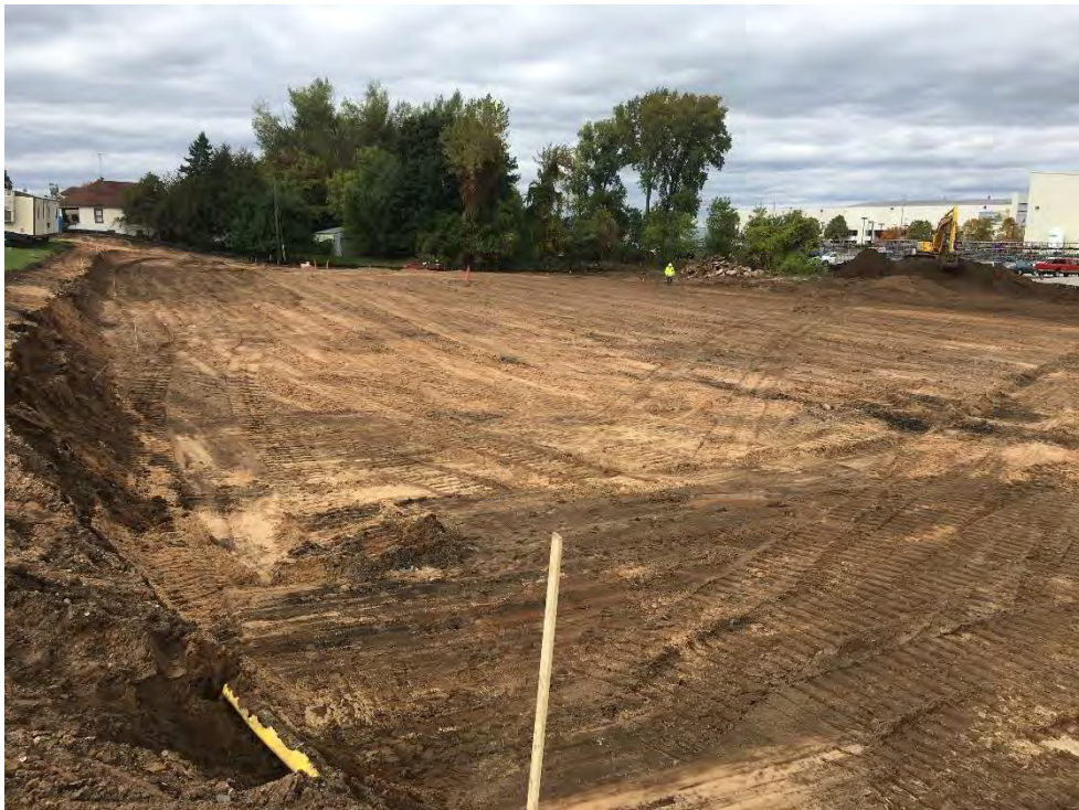
Photo 4 - Site stripped and regraded for building foundation; looking west
