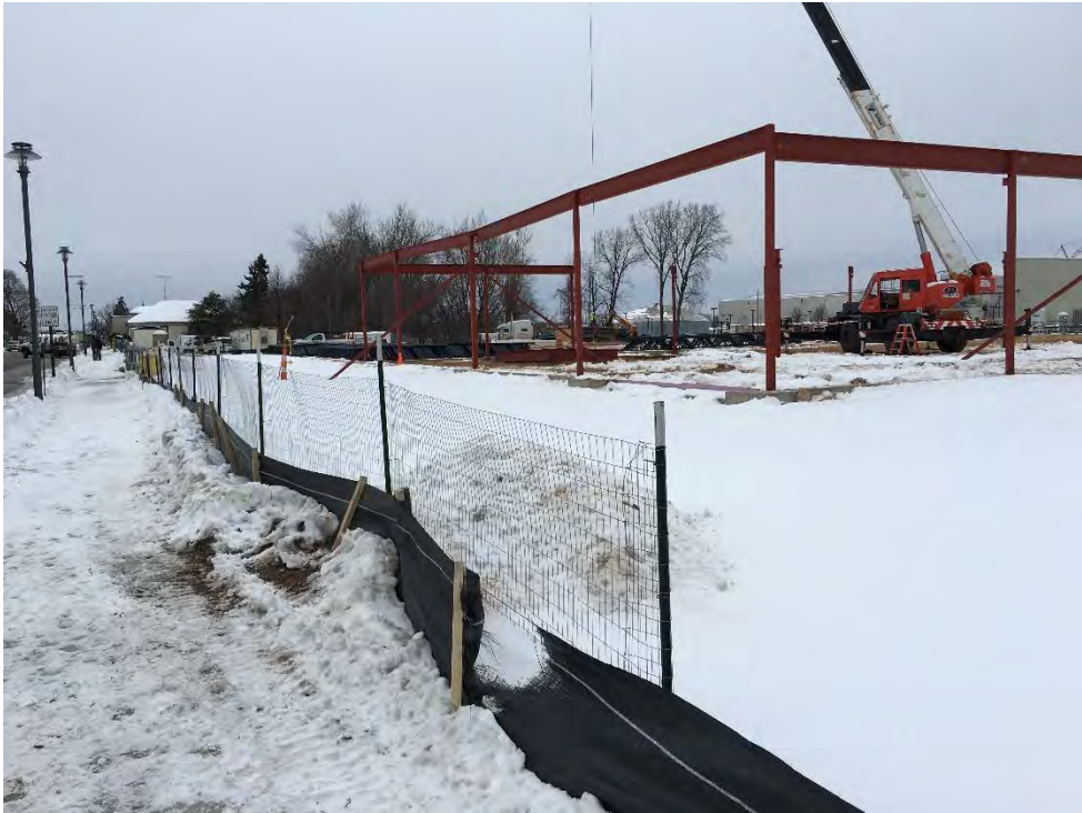
Photo 9 – Building construction; looking northwest
