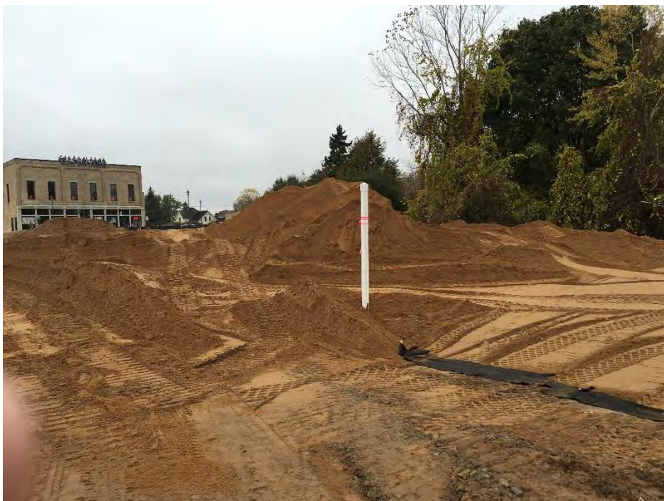
Photo 8 – Clean fill cap over filter fabric with MW1800; looking southwest
