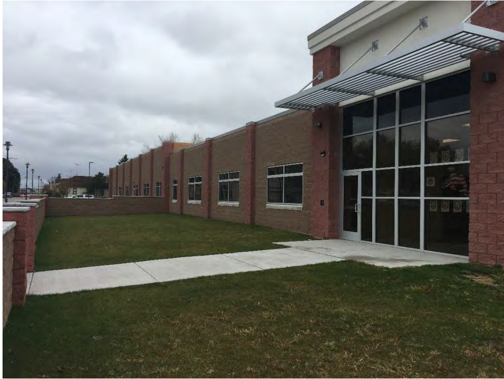
Photo 32 - Final site building; looking northeast across Main Street
