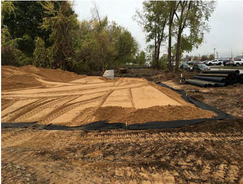
Photo 8 – Clean fill cap over filter fabric with MW1800; looking southwest
