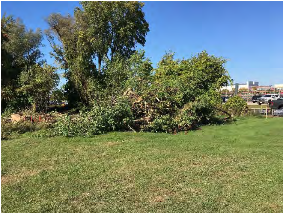
Photo 2 – Vegetation removal northwest corner of the Site; looking northwest
