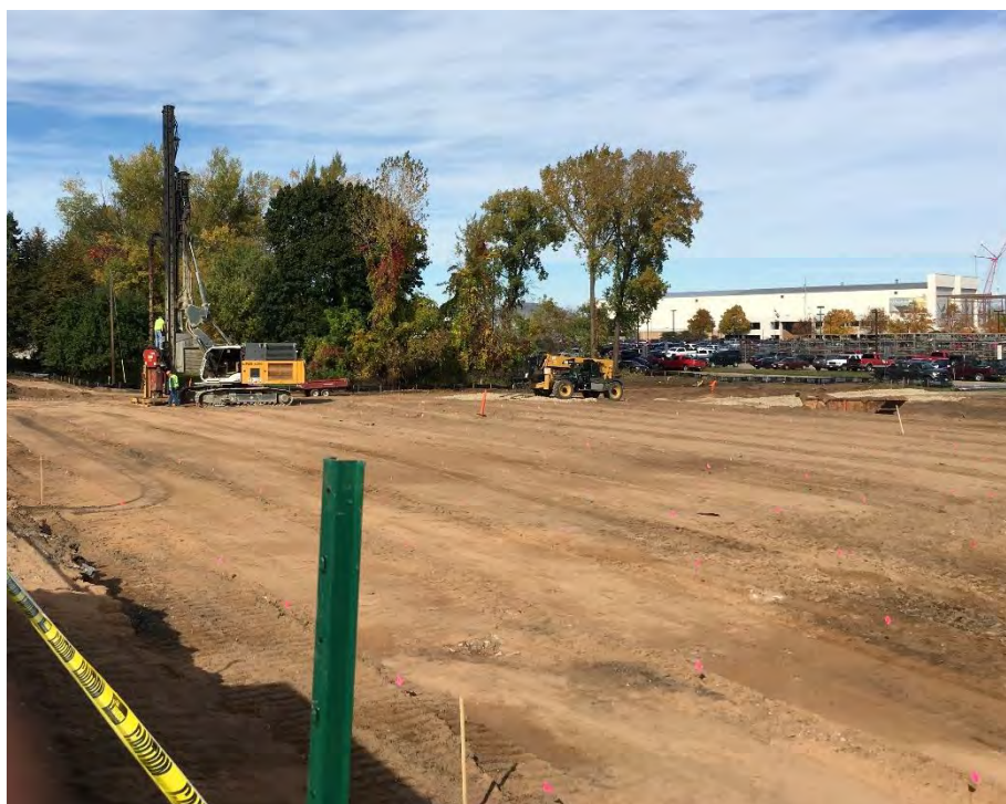
Photo 6 – Installation of geopiers; looking west
