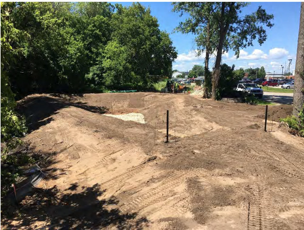
Photo 22 - Final clean soil cap over retention pond; looking northwest
