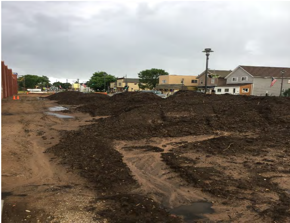
Photo 16 - Placement of topsoil; looking northwest along Ludington Street
