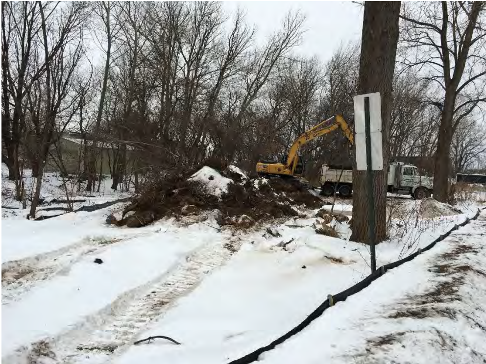
Photo 10 – Retention pond construction/excavation; looking northwest
