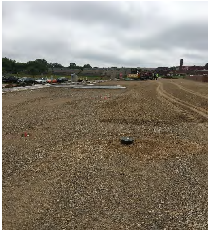
Photo 18 - Placement of gravel subgrade in parking lot; looking southwest
