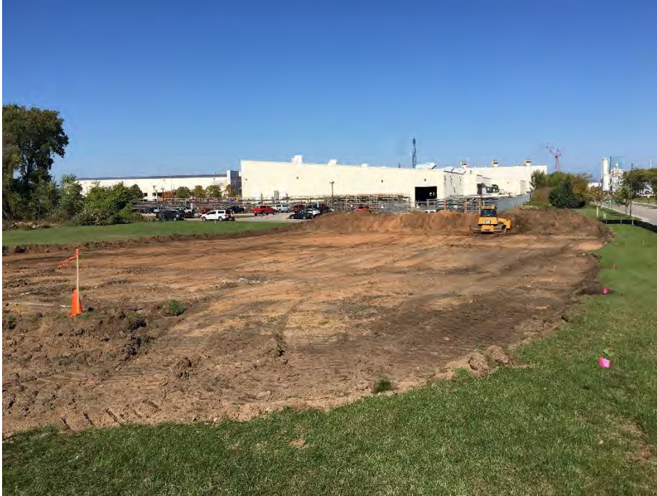
Photo 1 – Topsoil and vegetation stripping; looking north
