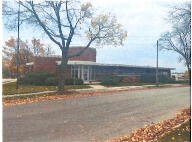
IMAGE 3: VIEW SOUTHEAST OF AMCAST SOUTH, SHOWING THE OFFICE BUILDING.
