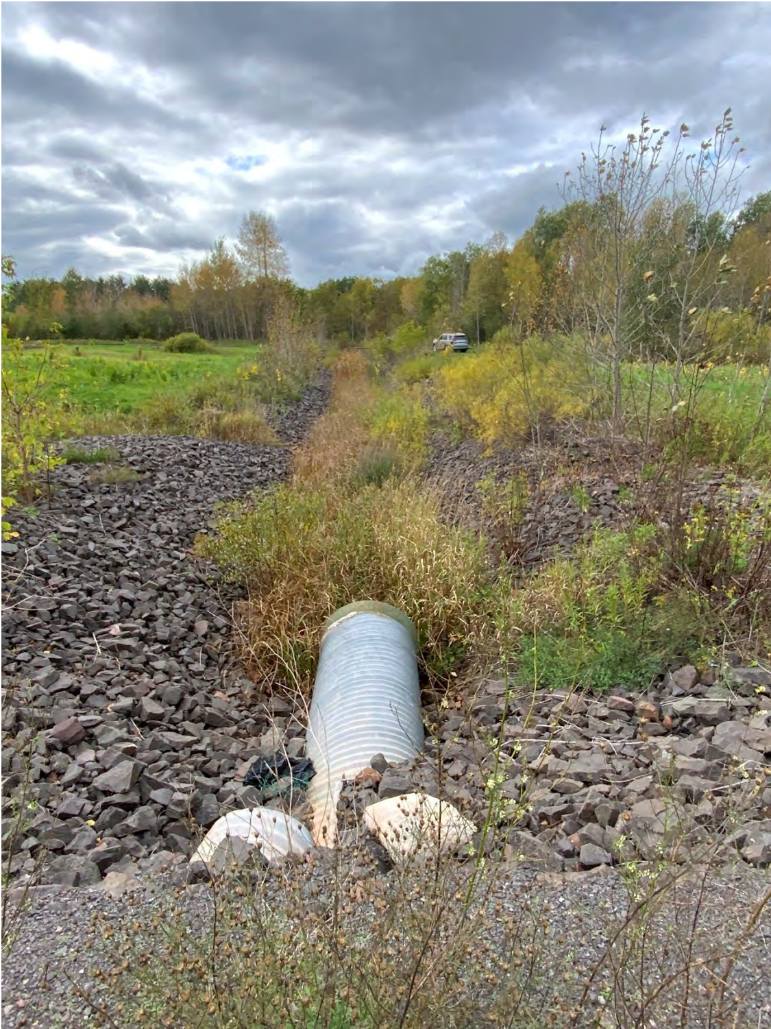
Outfall 001 Drainage Ditch Photo 1, looking West from Eastern edge:
